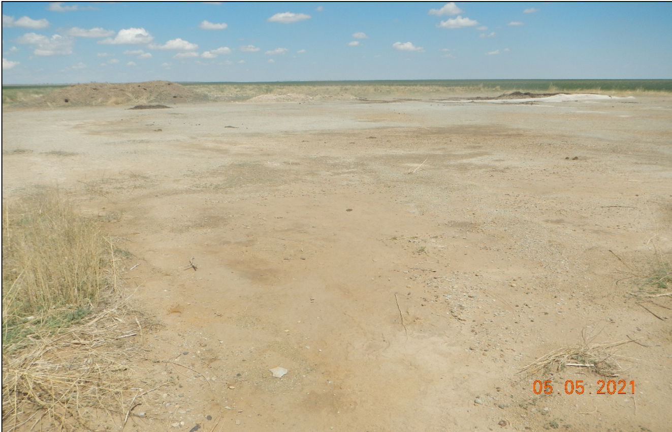
Photo 2. Facing north toward the location. Soils are compacted and the location has not been reclaimed. Previous corrective actions were not performed. Soils must be decompacted by cross ripping to a depth of 18 inches.
