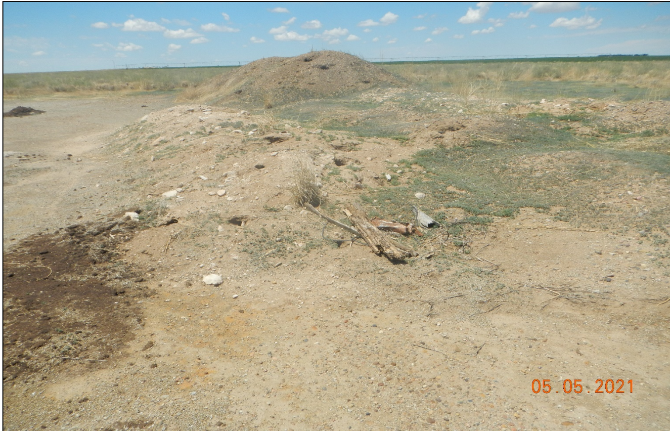
Photo 6. There are gravel and soil piles that remain at the northwest side of the location. The piles need to be removed. There are undesirable weeds growing on the piles.
