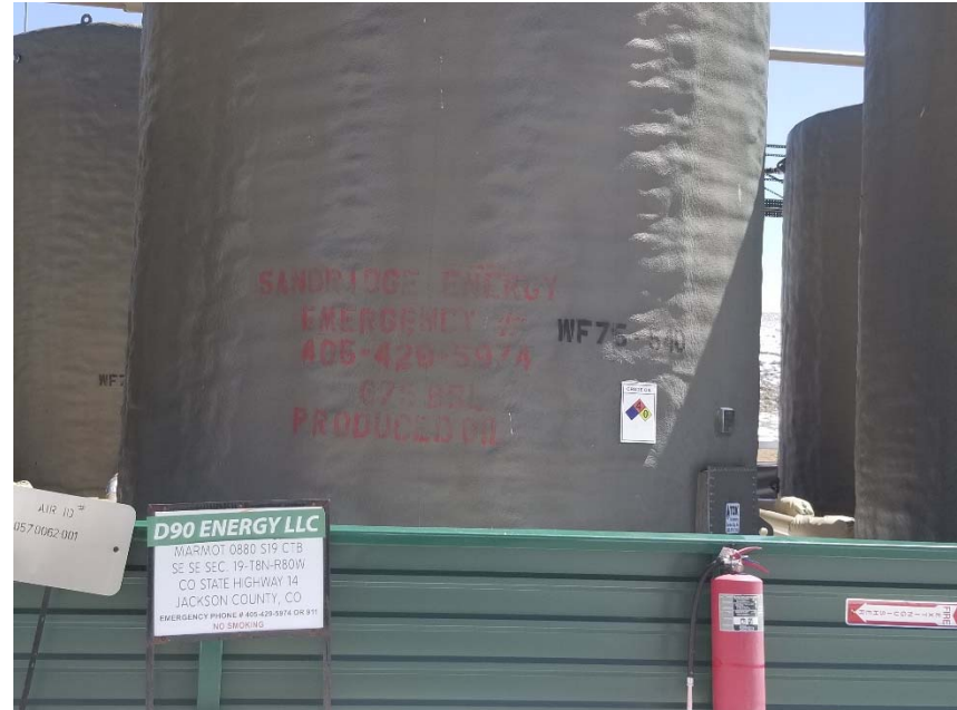
Photo 4. Incomplete and inaccurate tank labels and battery sign.
