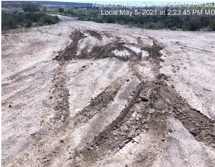
Photo #3727 No form of tracking BMP at entrance to location.
