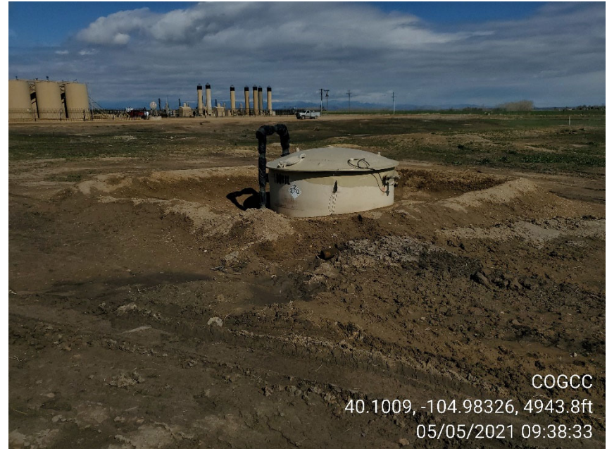
Photo 2 Produced water vessel containment requiring maintenance.
