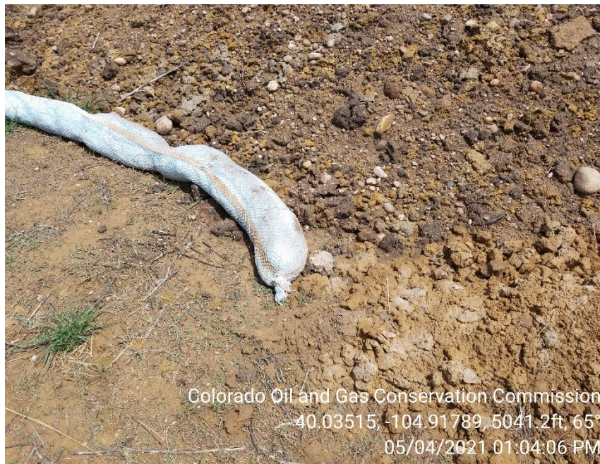
Photo 9 – Soils stored on location with inadequate BMPs
