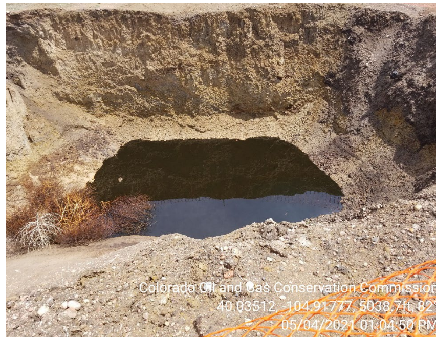
Photo 4 – Open excavation. Free product observed on groundwater. Impacts remain in situ.
