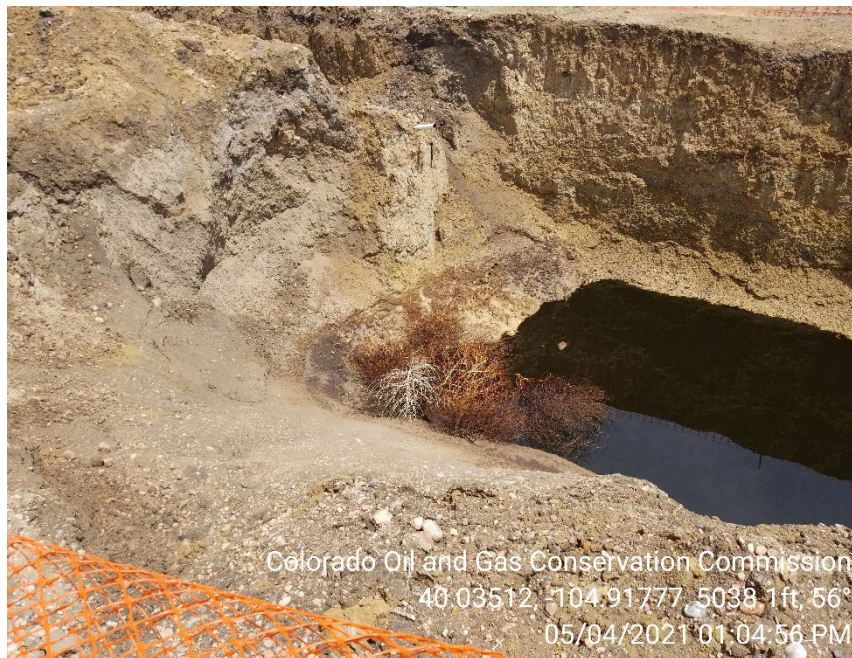
Photo 3 – Open excavation. Free product observed on groundwater. Impacts remain in situ.
