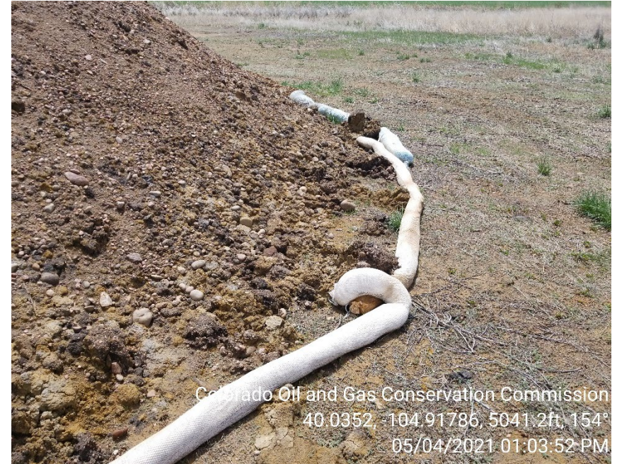
Photo 8 – Soils stored on location with inadequate BMPs
