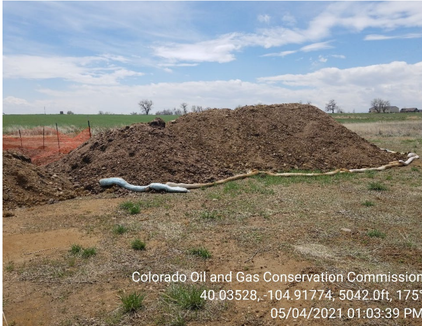
Photo 7 – Soils stored on location with inadequate BMPs
