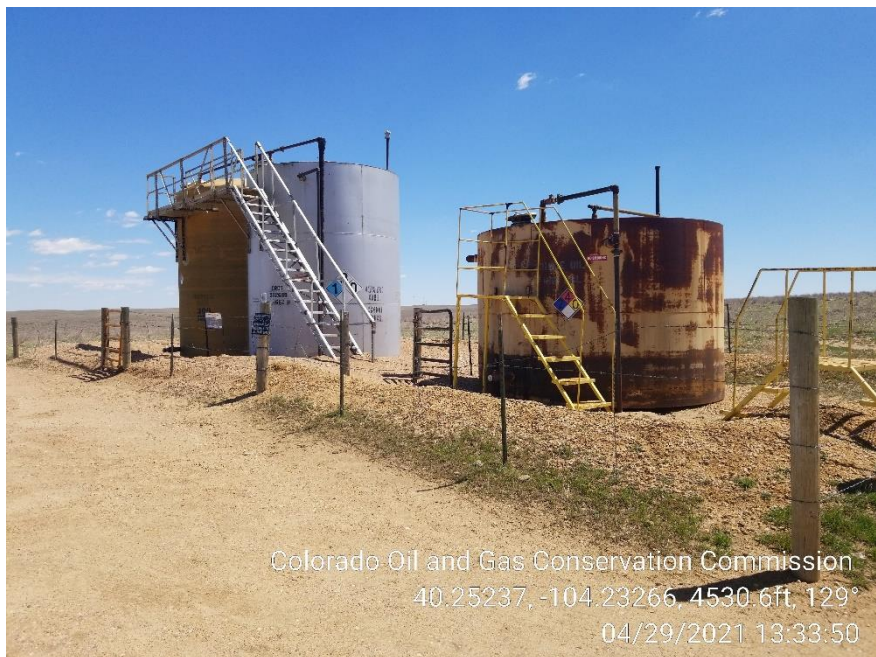
Photo 3 – Tank Battery – Weeds. Produced Water Content Label Fading
