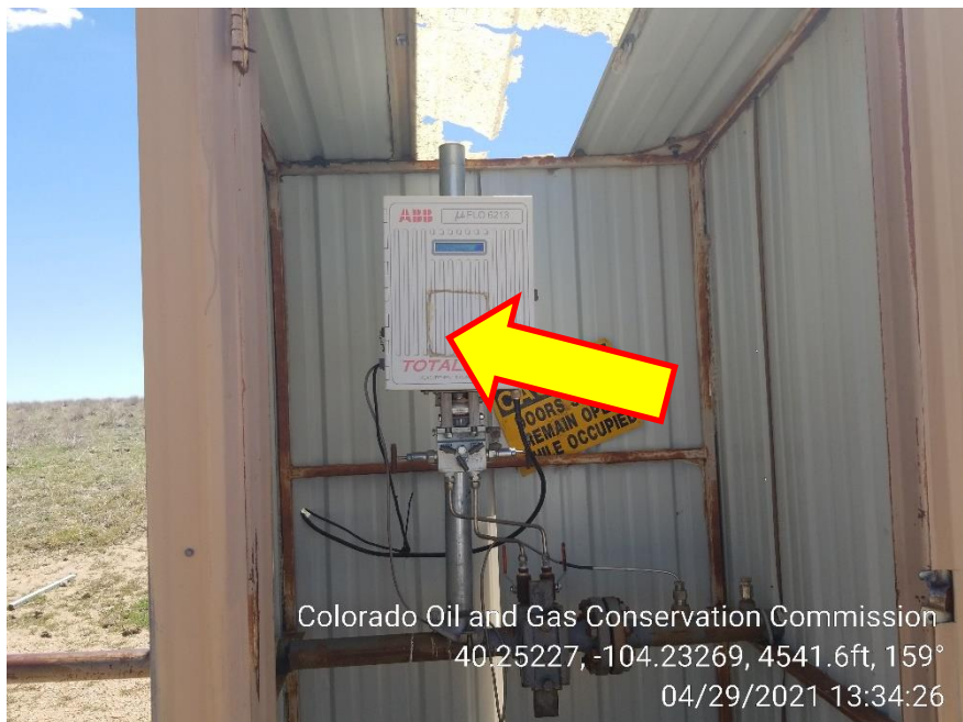
Photo 5 – Gas Meter Calibration Card missing
