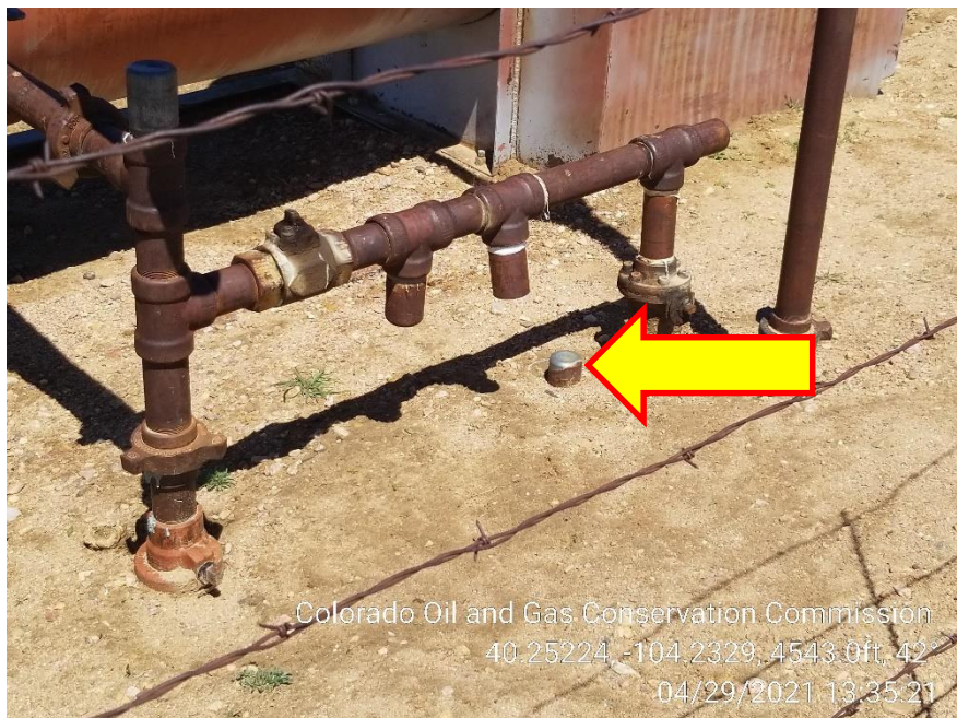
Photo 7 – Unmarked Riser at Separator
