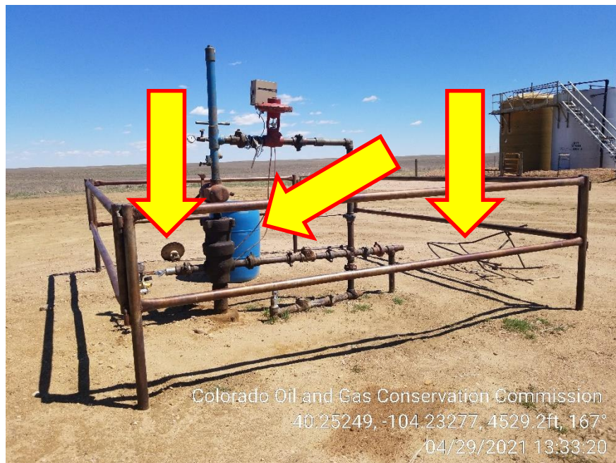
Photo 1 – Wellhead – Unused Motor Valve, Chemical Tank and Stand
