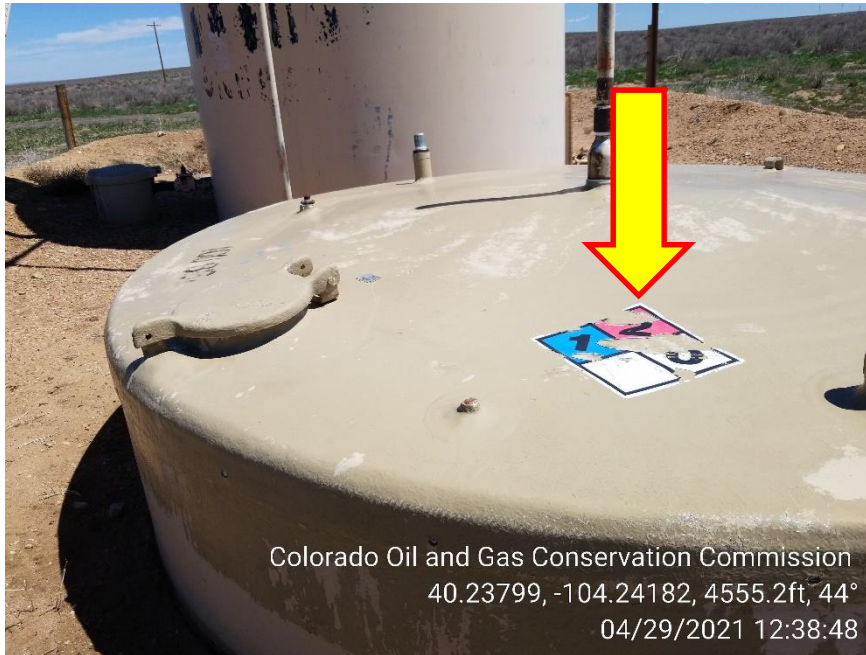
Photo 5 – NFPA Label is fading
