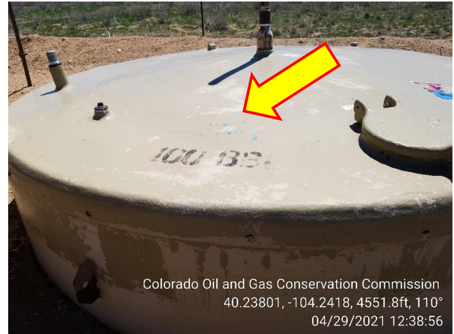
Photo 6 – Content Label is missing
