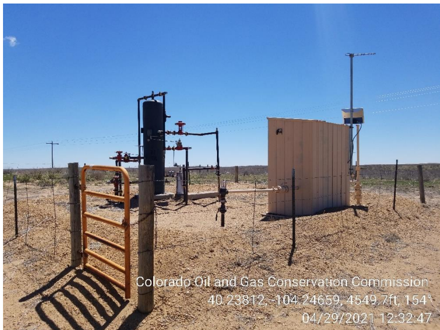
Photo 5 – Gas Meter Shed and Separator
