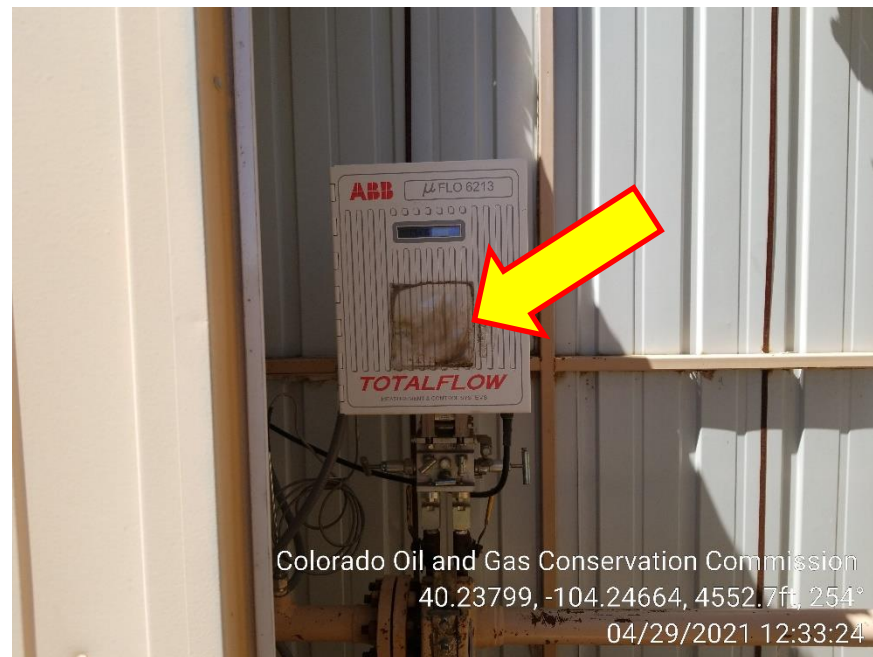
Photo 6 – Gas Meter Calibration Card NOT Present
