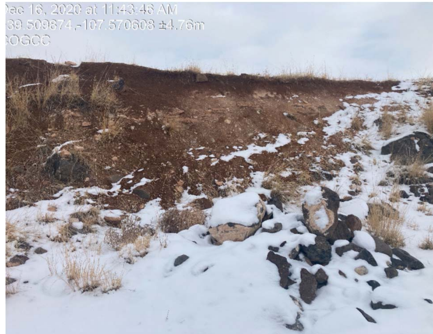
Previous inspection photo of lack of stabilization/erosion
