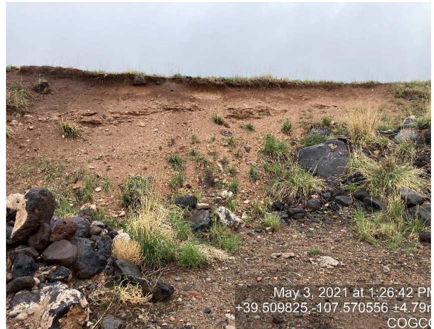
Follow up inspection photo of lack of stabilization/erosion
