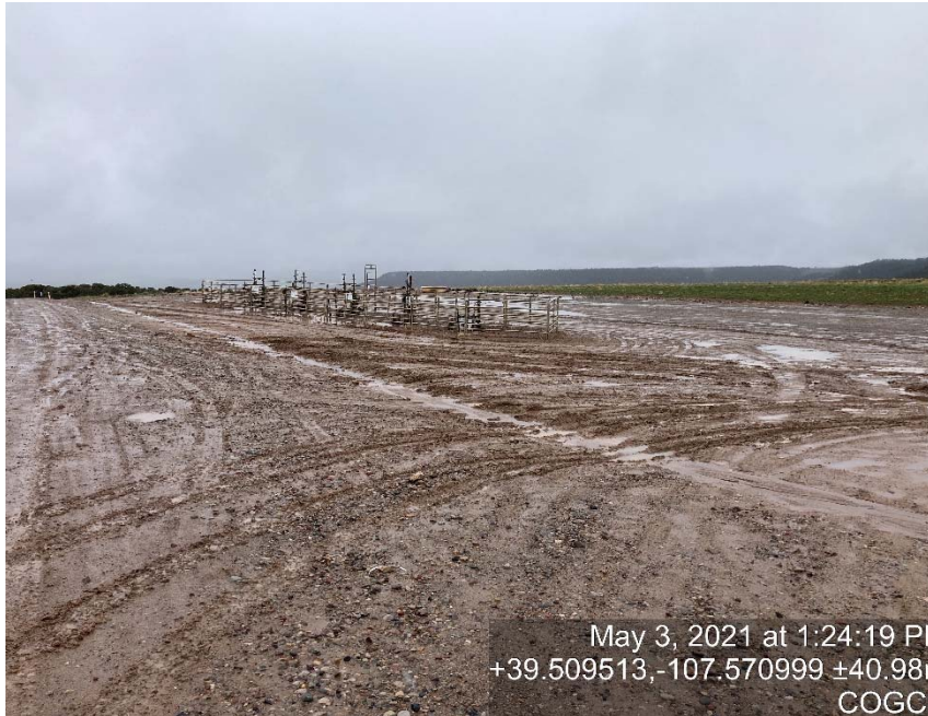
Location/Lack of stabilization/ compaction/tracking
