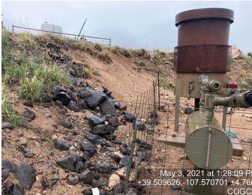
Lack of stabilization/erosion
