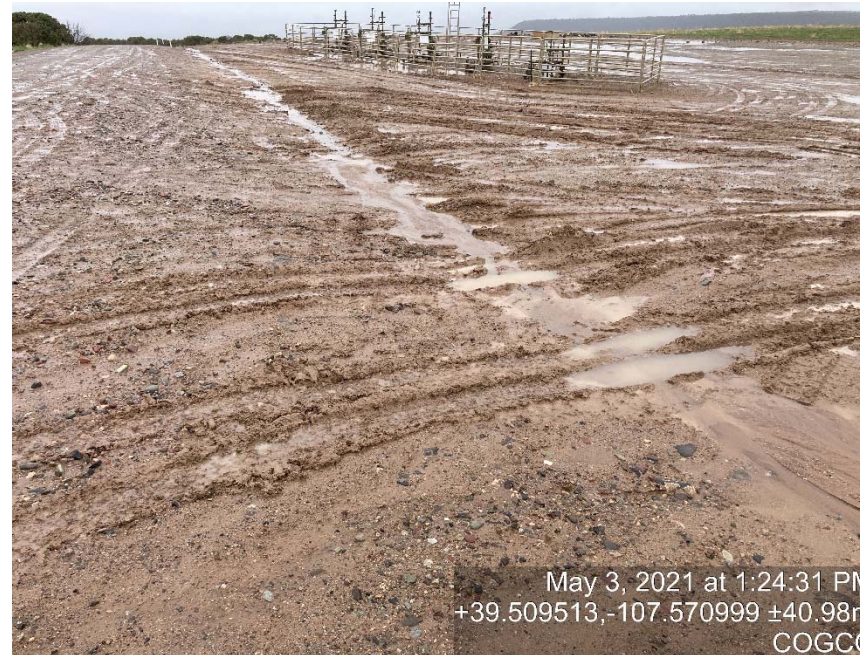
Lack of stabilization/ compaction/tracking
