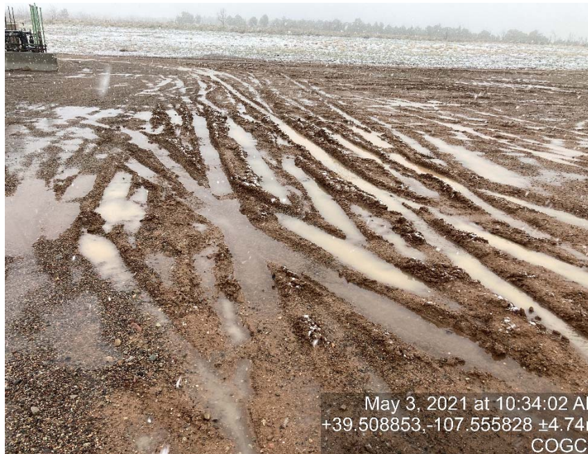
Lack of stabilization/compaction
