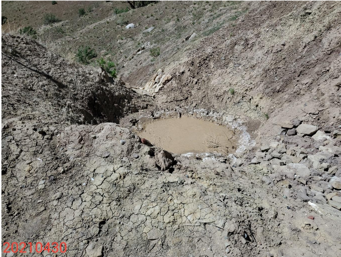
Photo 1: Photo shows sediment trap on the southwest corner of the Location. Sediment trap observed to not have been installed with geotextile lining in accordance with good engineering practices; soils observed to be eroding beneath the rock arming at the inlet/outlet
