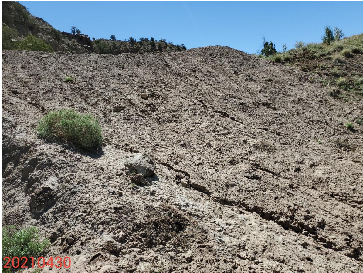
Photo 7: Photo taken from the northeastern slopes of the Location, facing east. Previous inspections required Operator to implement control measures to stabilize and protect the slopes of the Location. Photo shows control measures remains missing or insufficient to stabilize and protect slopes.
