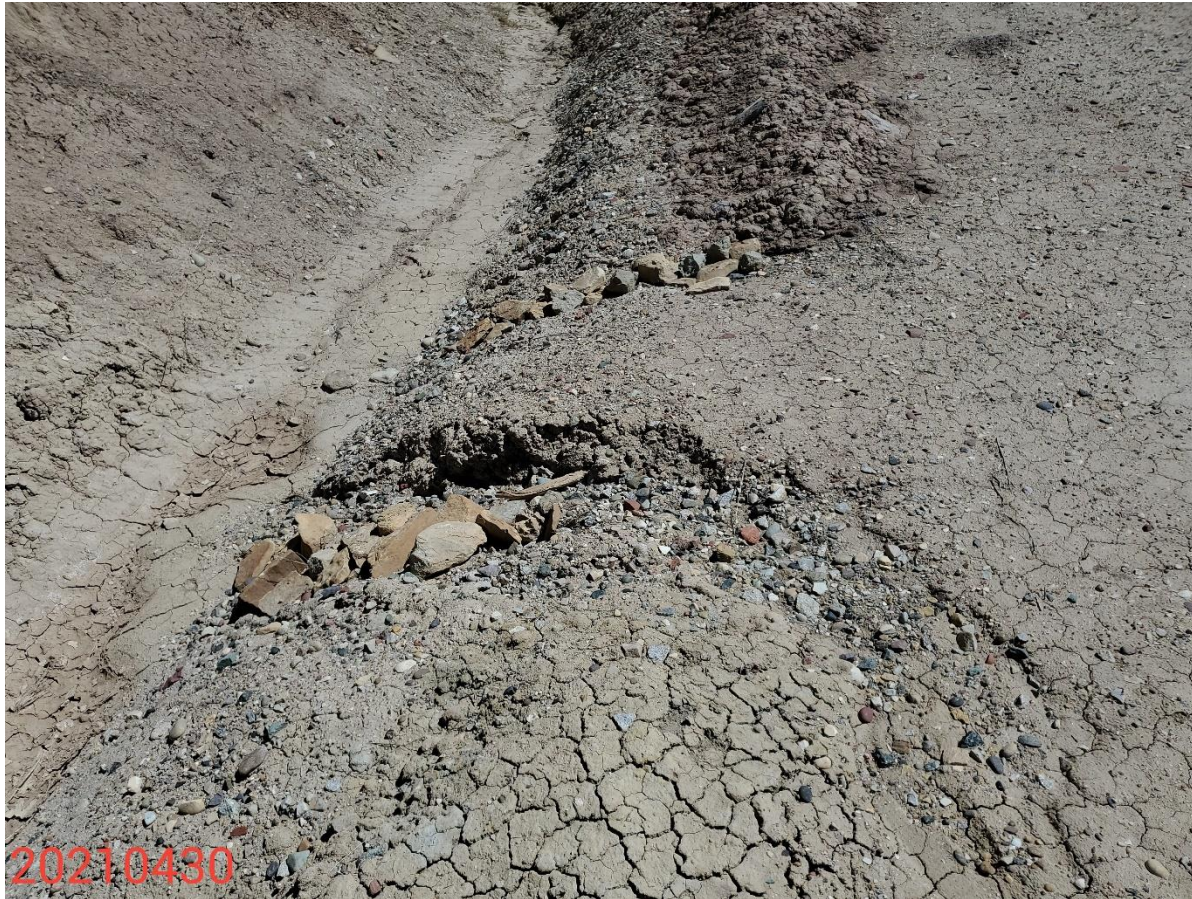
Photo 5 Photo taken from the ditch. Photo shows example of areas observed along the ditch, where rock armoring was placed to mitigate degradation and protect ditch/location; control measures inadequate to prevent degradation.
