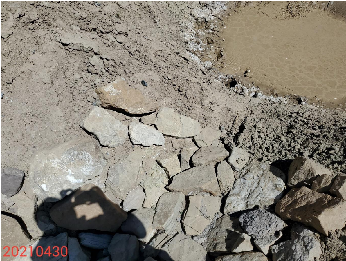
Photo 2: See comments under photo 1. Soils observed to be eroding beneath the rock armoring.
