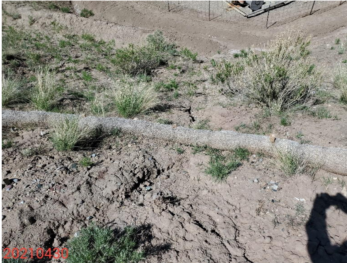
Photo 8: See comments under photo 6. Photo also shows stormwater movement will travel beneath the wattle within the gully.
