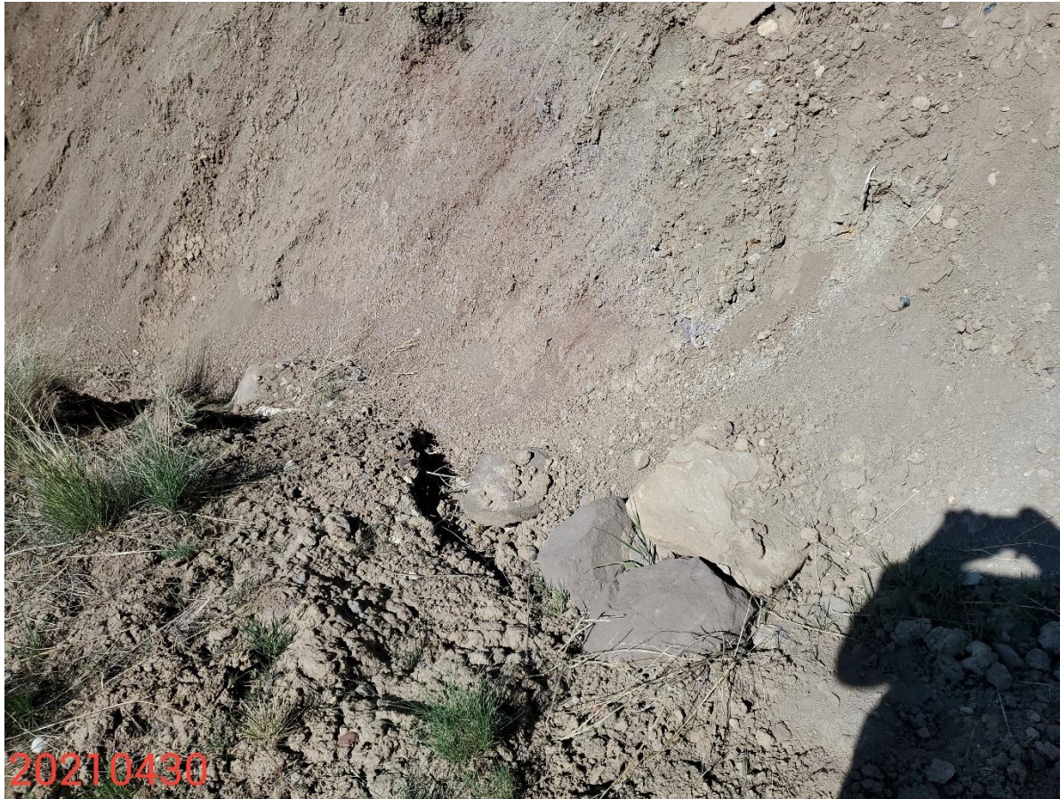
Photo 3: See comments under photo 1. Soils observed to be eroding beneath the rock armoring.
