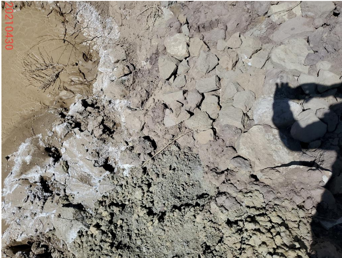
Photo 4: See comments under photo 1. Soils observed to be eroding beneath the rock armoring.
