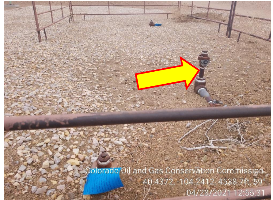
Photo 6 – Riser Tag/Marked Missing
