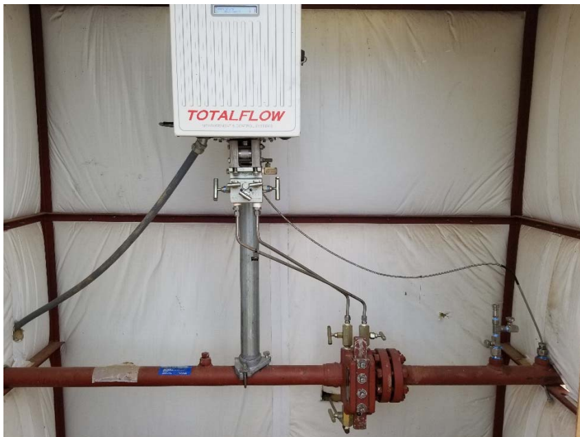
Photo 2. No calibration information in meter run.
