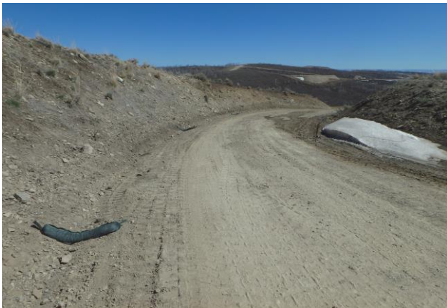
Bar Ditch Installed below Eastern Cut-Slope
