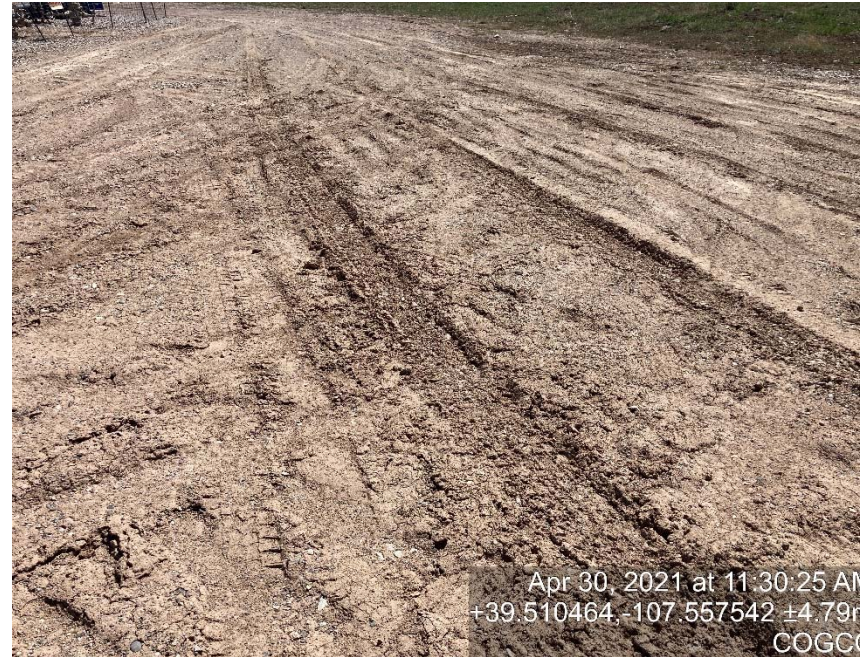
Lack of stabilization/compaction
