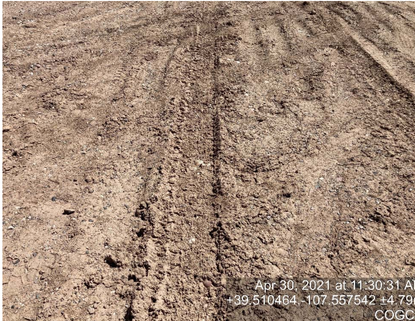
Lack of stabilization/compaction
