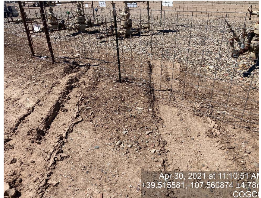
Lack of stabilization/compaction
