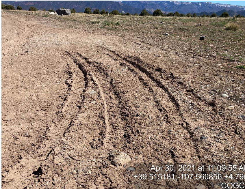
Lack of stabilization/compaction
