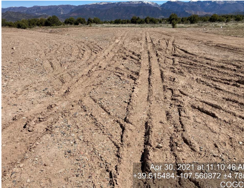
Lack of stabilization/compaction
