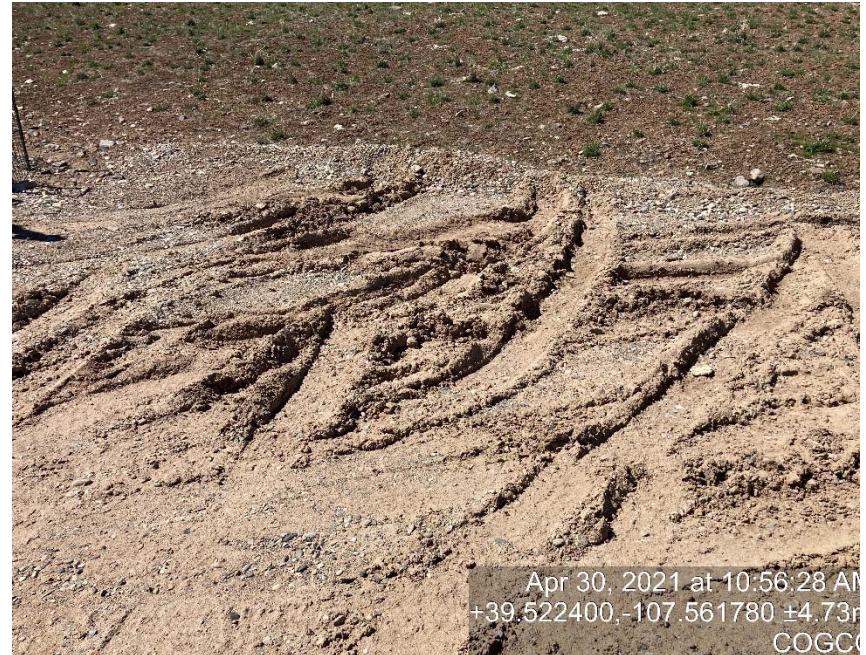
Lack of stabilization/compaction
