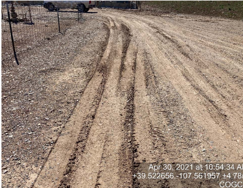
Lack of stabilization/compaction
