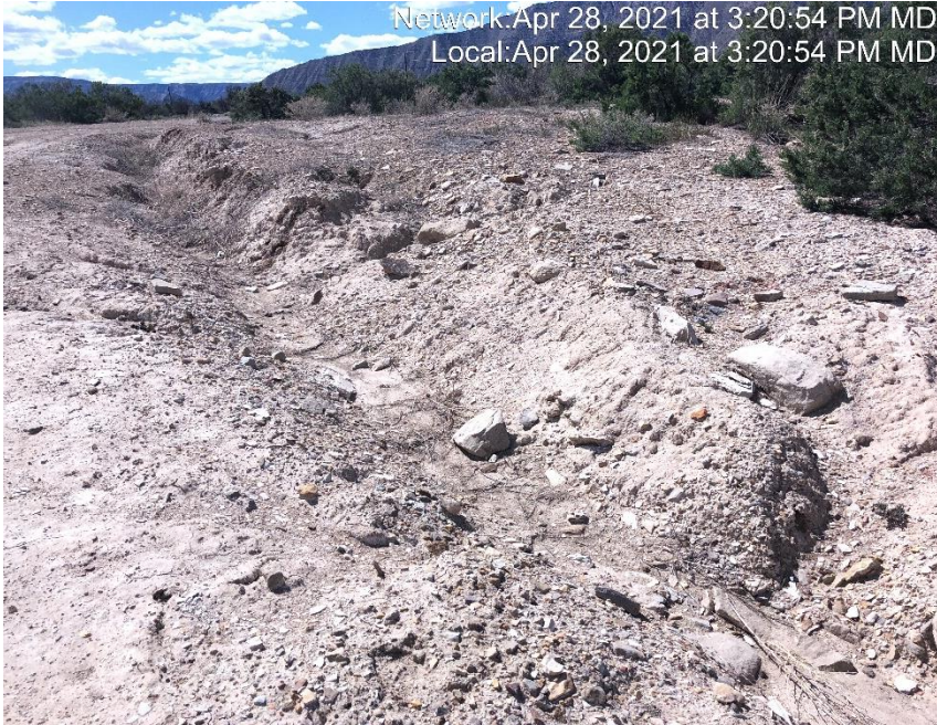
Photo #3668 No velocity checks.
