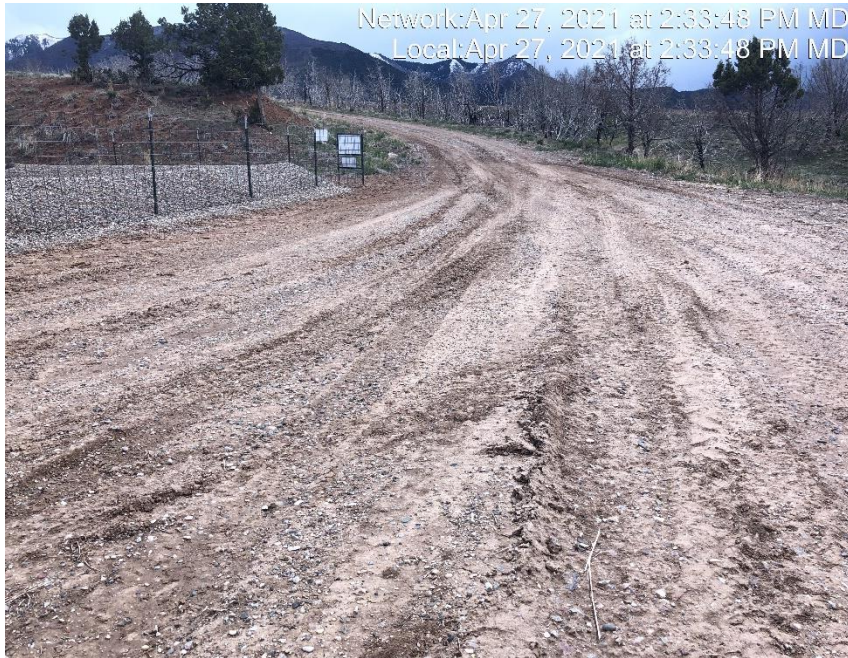
Photo #3646 No form of Tracking BMP at entrance to location.
