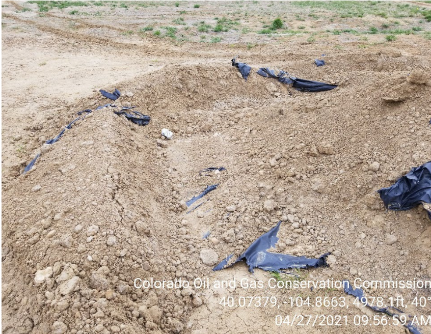
Photo 5 – Oily soils stockpiled on location. Lining does not adequately protect surface soils.
