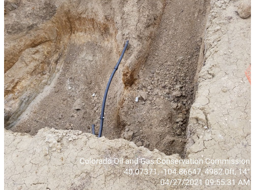
Photo 2 – Spill excavation. Impacts remain in situ. Trash observed in open excavation.
