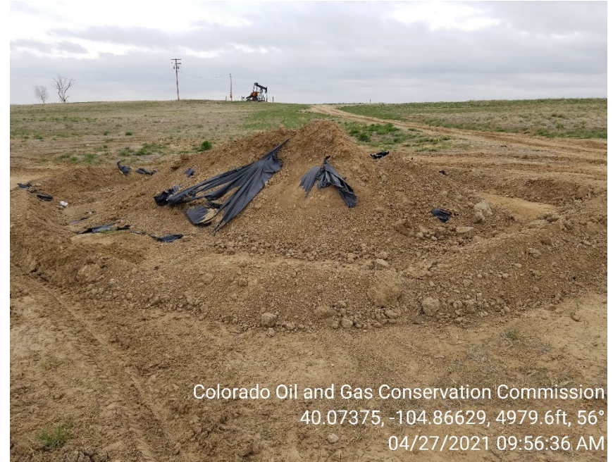
Photo 6 – Oily soils stockpiled on location. Lining does not adequately protect surface soils.
