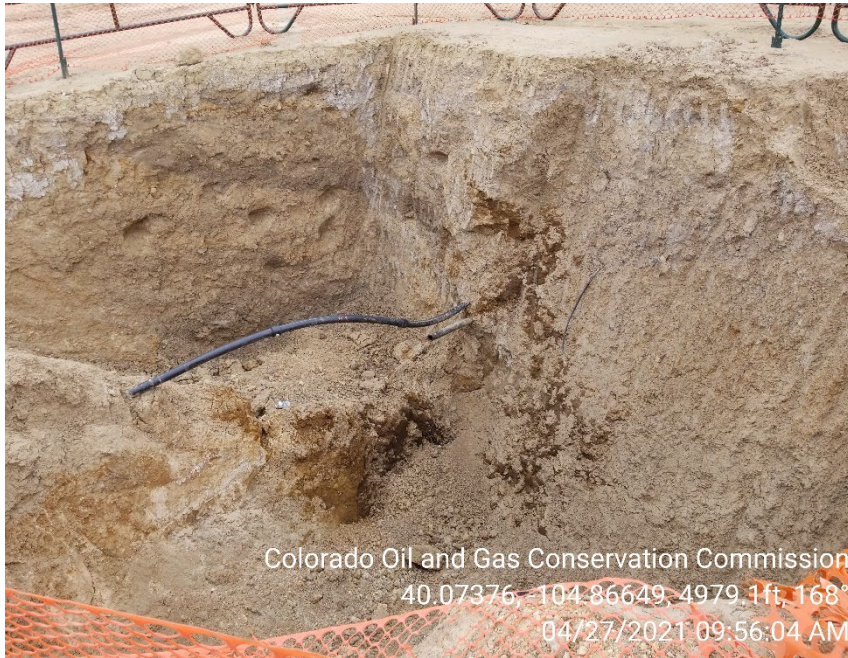
Photo 3 – Spill excavation. Impacts remain in situ. Trash observed in open excavation.
