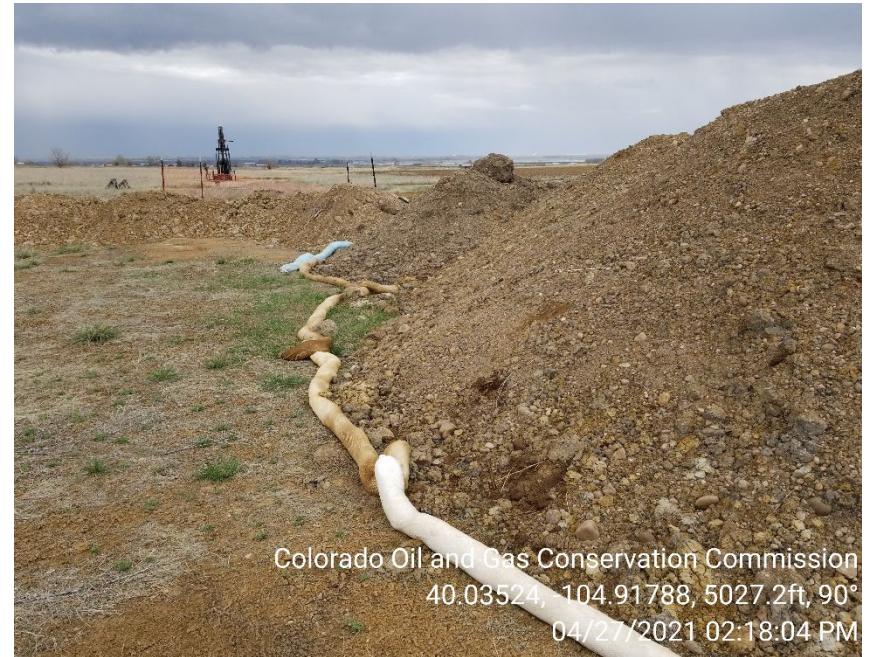
Photo 10 – Soils stored on location with inadequate BMPs
