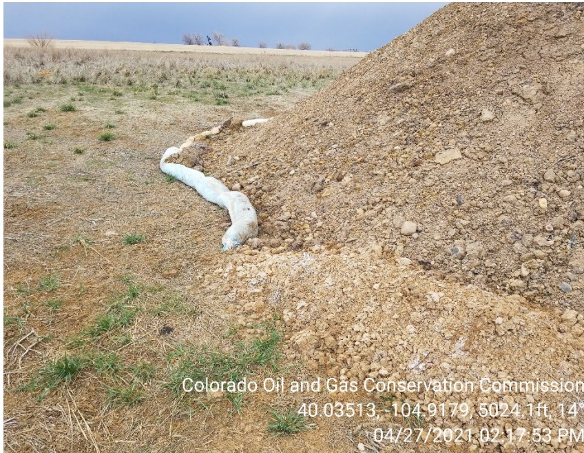
Photo 9 – Soils stored on location with inadequate BMPs
