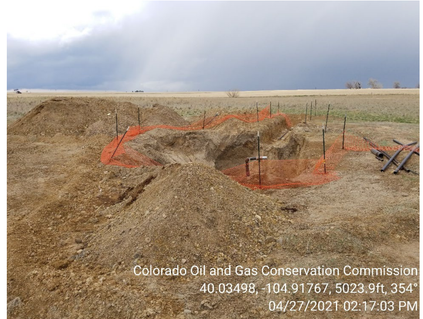
Photo 2 – Spill area. Fencing down around open excavation. Soils stockpiled on location. Trash on location.
