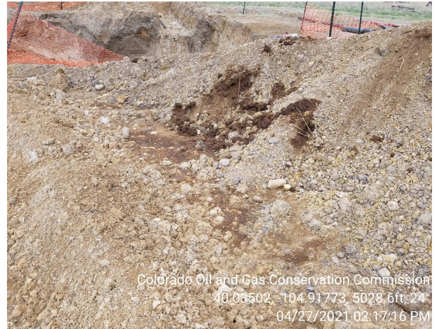
Photo 6 – Impacted soils remain on surface outside of excavation area. Soils stockpiled on location with inadequate BMPs.
