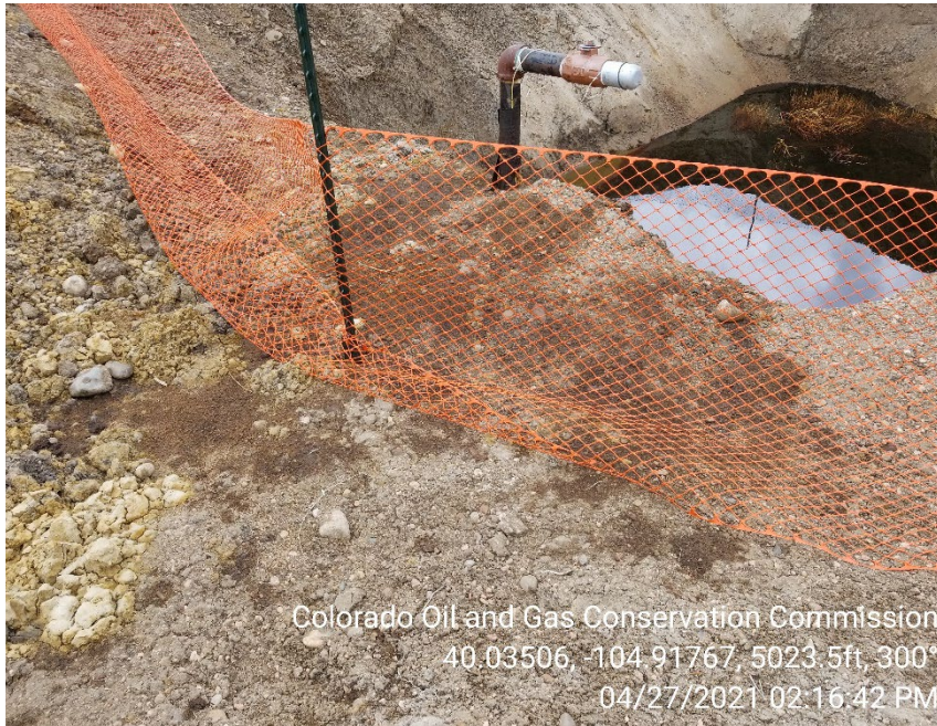
Photo 5 – Impacted soils remain on surface outside of excavation area.
