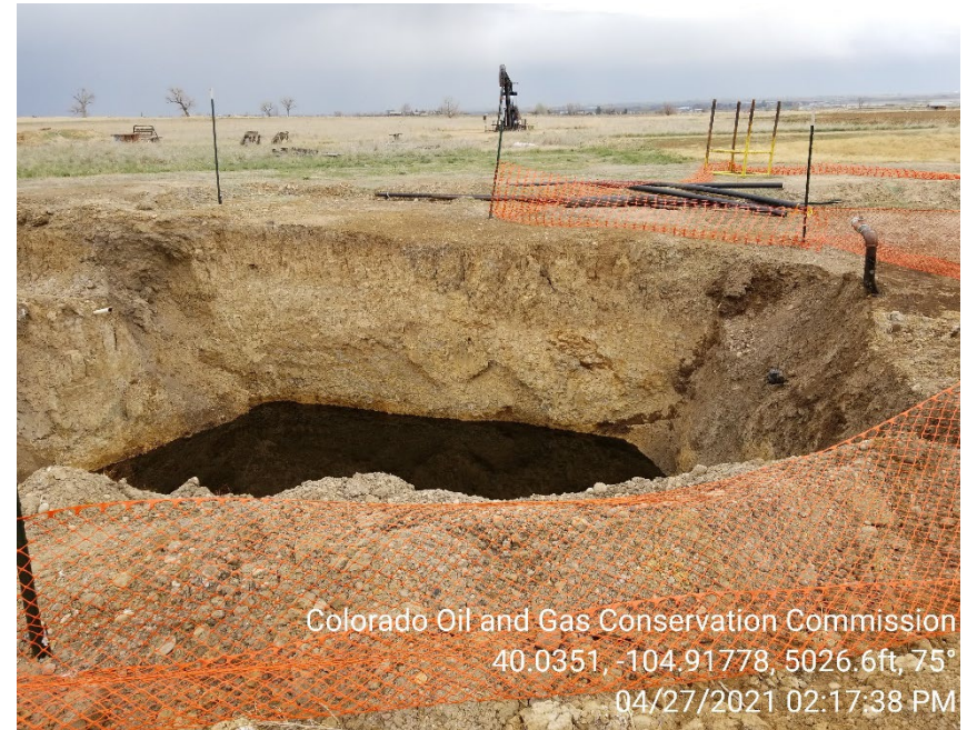
Photo 4 – Open excavation. Free product observed on groundwater. Impacts remain in situ.
