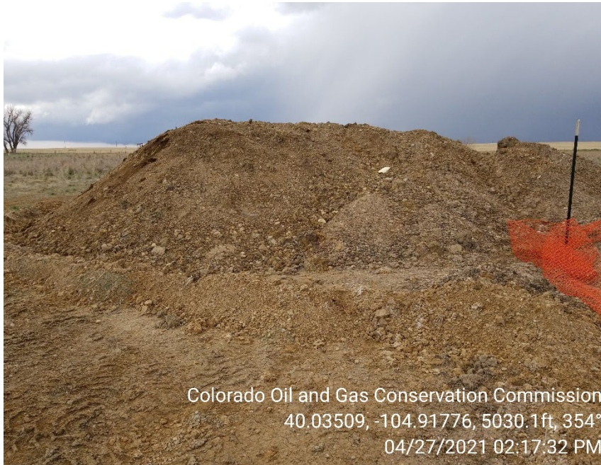
Photo 7 – Soils stored on location with inadequate BMPs
