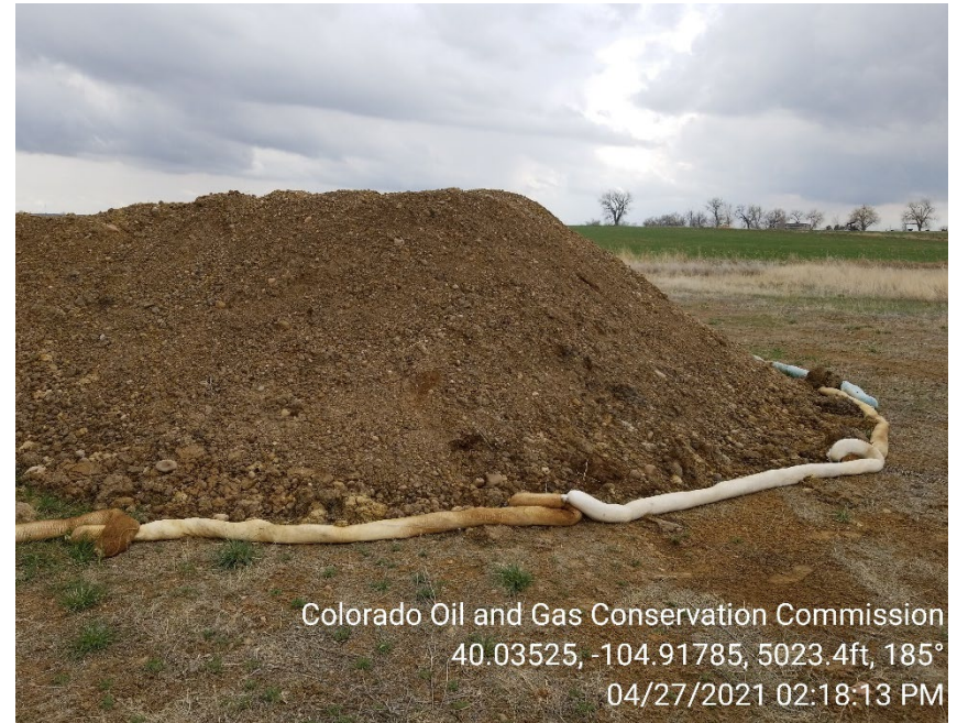
Photo 8 – Soils stored on location with inadequate BMPs
