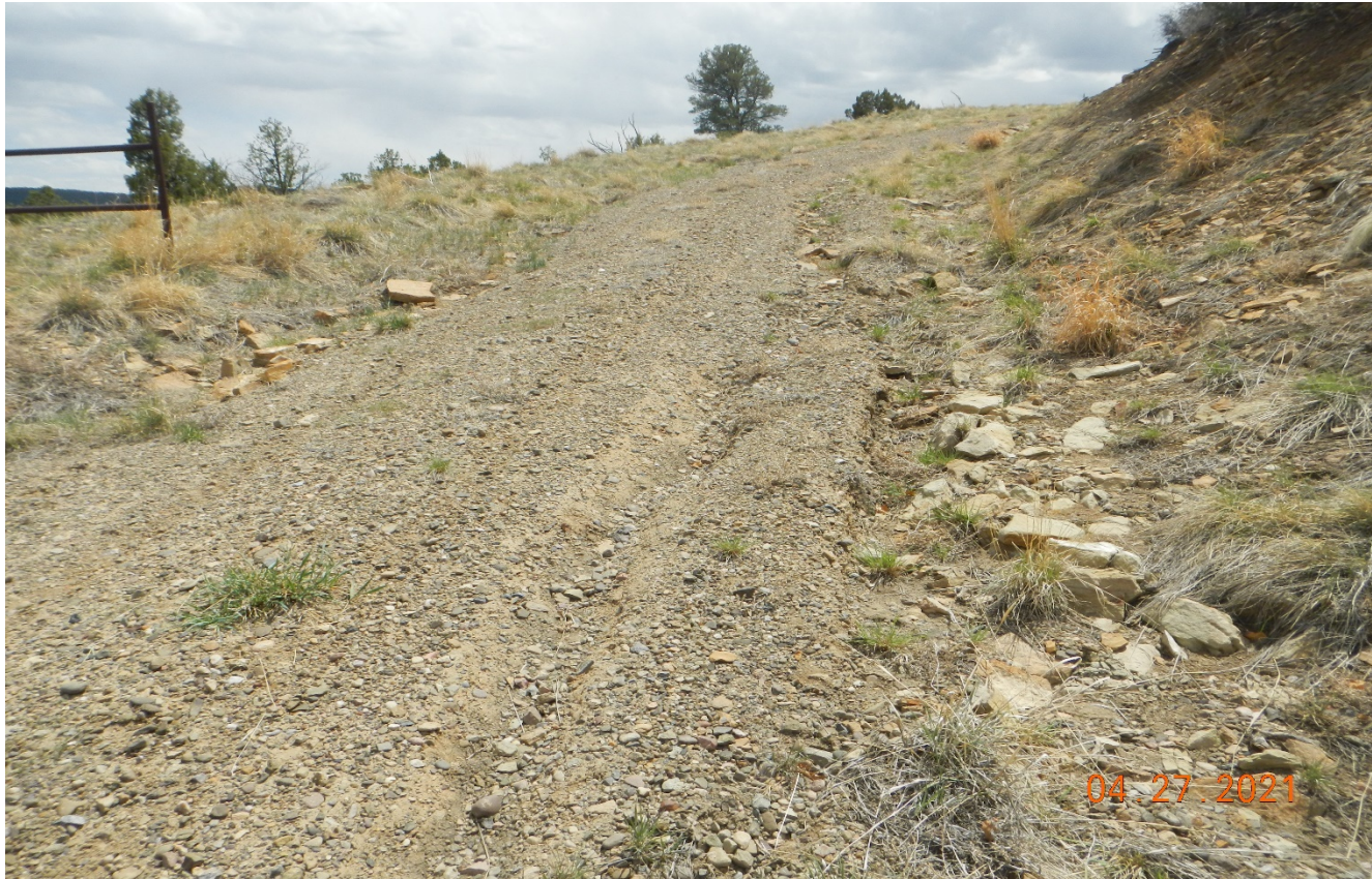
Photo 2. Facing south along the access road. The road has not been recontoured and reclaimed. There are signs of stormwater erosion down the road.
