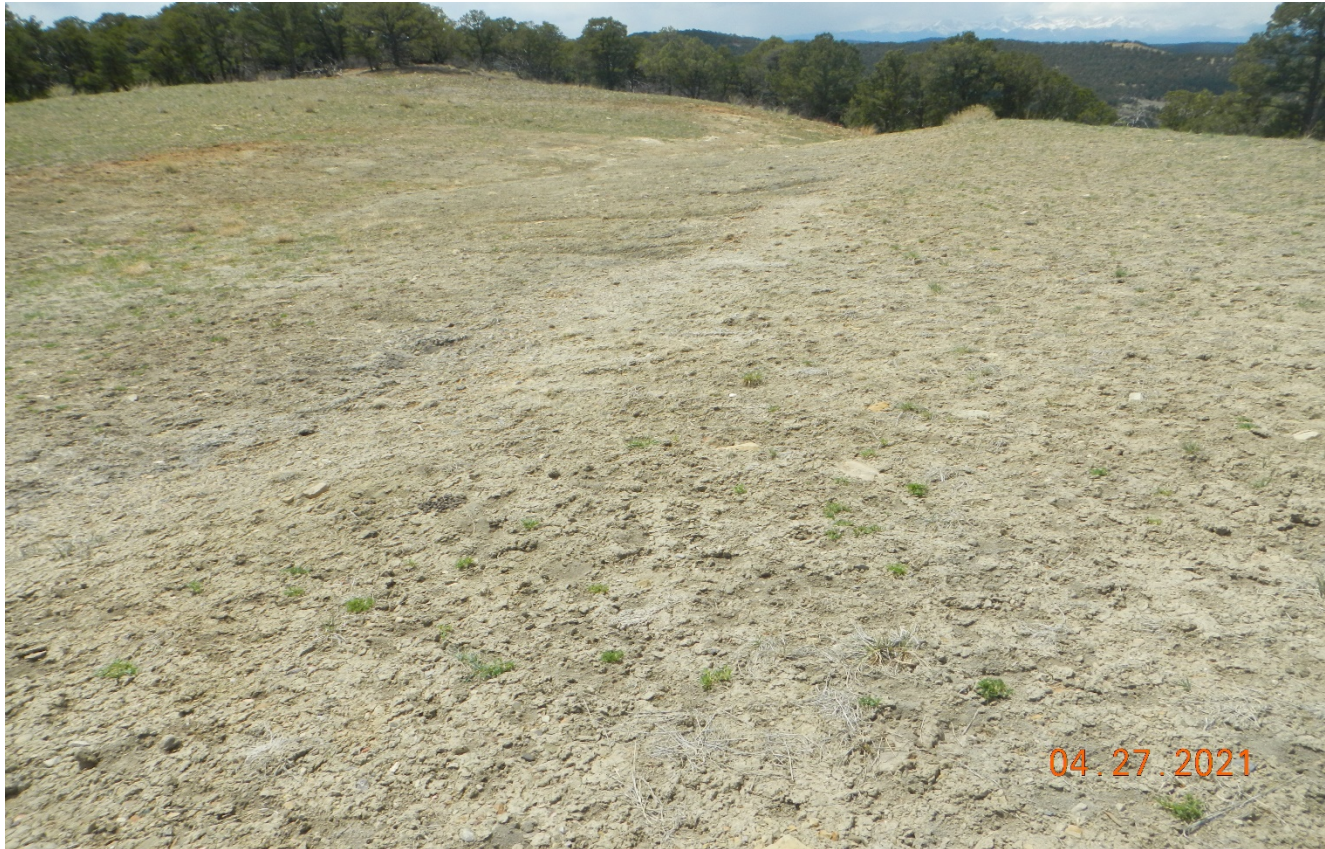
Photo 5. Facing west at the location. The soils are not stabilized and are susceptible to erosion. BMP's have not been installed.
