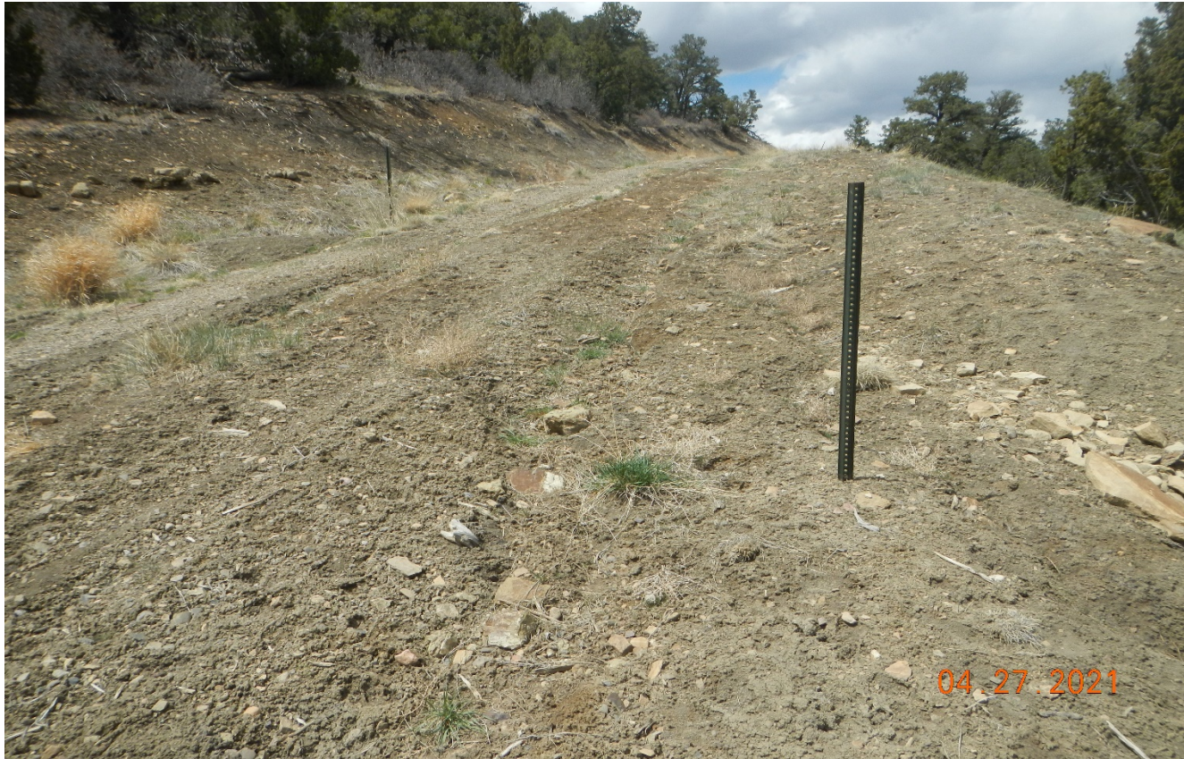
Photo 1. Facing northwest the beginning of the access road. The road has not been recontoured and reclaimed. There are signs of stormwater erosion down the road.
