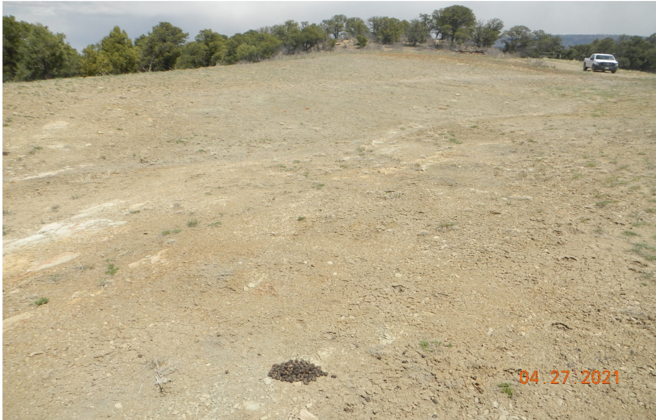
Photo 6. Facing northeast at the location. The location is not stabilized and there are signs of erosion. BMP's have not been installed.
