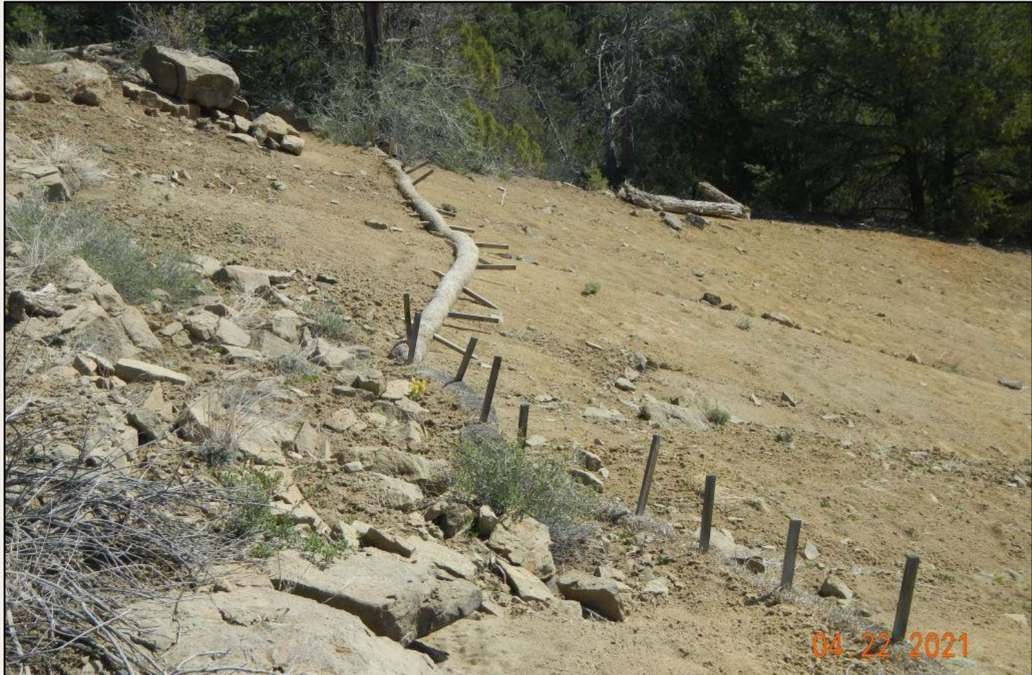
Photo 4. View of wattles at the top of the eastern cut-slope that need maintenance. Erosion controls (ie jute mat, straw blanket, etc. are needed to stabilize blare soils on the cut-slope. Care needs to be take to prevent damage to desirable perennial vegetation.
