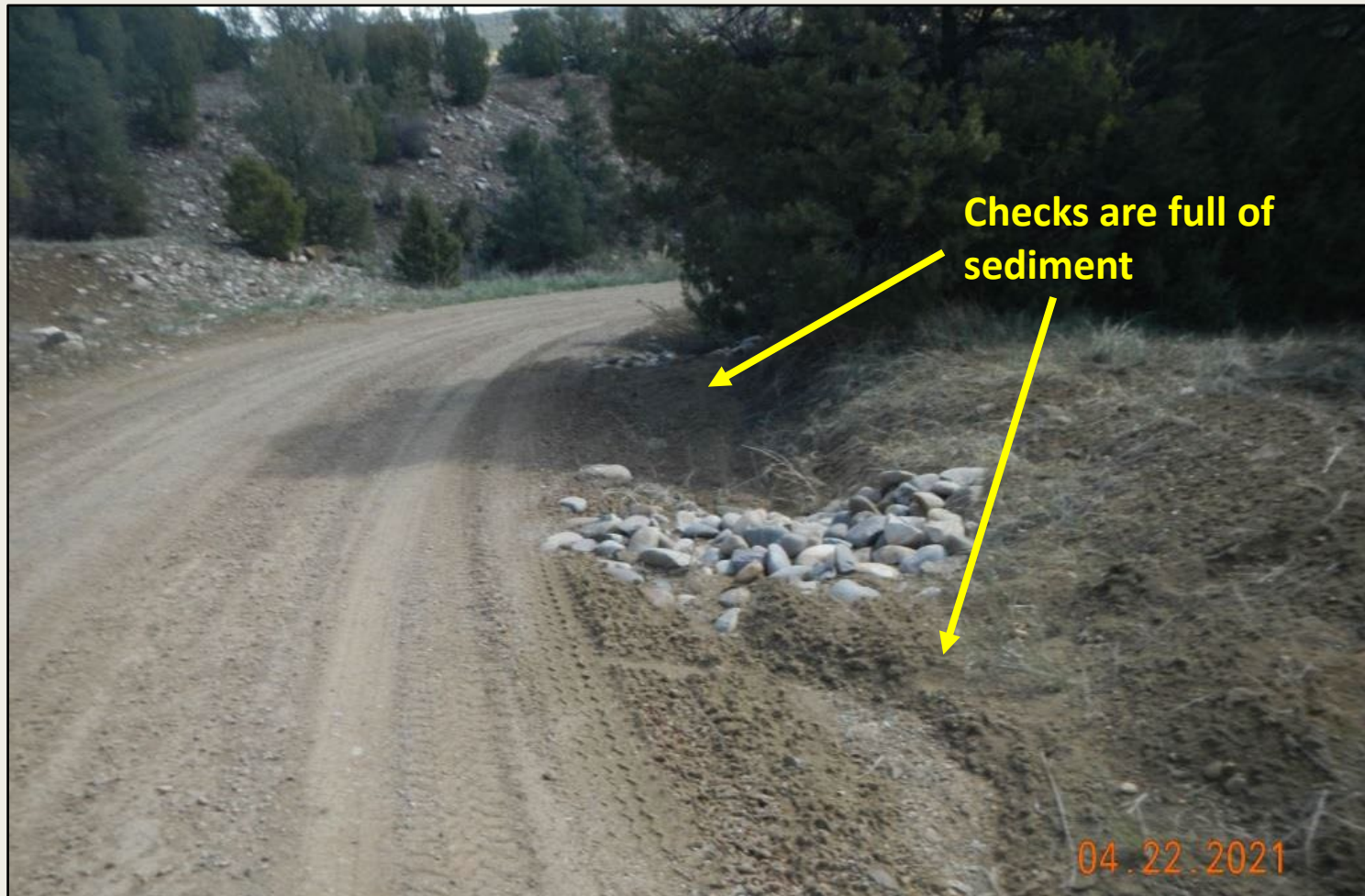
Photo 3. View of rock velocity checks along the access road that are full of sediment and are not adequate BMPs for this slope.
