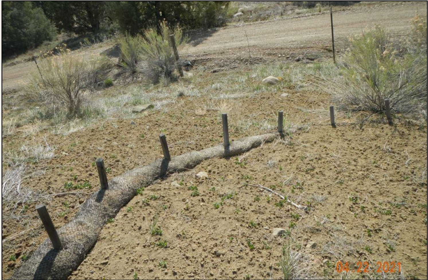
Photo 5. View of wattle in the southeastern project area, that is full of sediment and needs maintenance.
