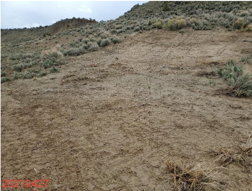
Photo 1: Photo taken from the Location, facing south. Photo shows areas where work to remove stained soils was previously conducted. Photo shows requires stormwater and erosion control remain missing or insufficient. Unable to find evidence that seeding/revegetation activities have been performed.
