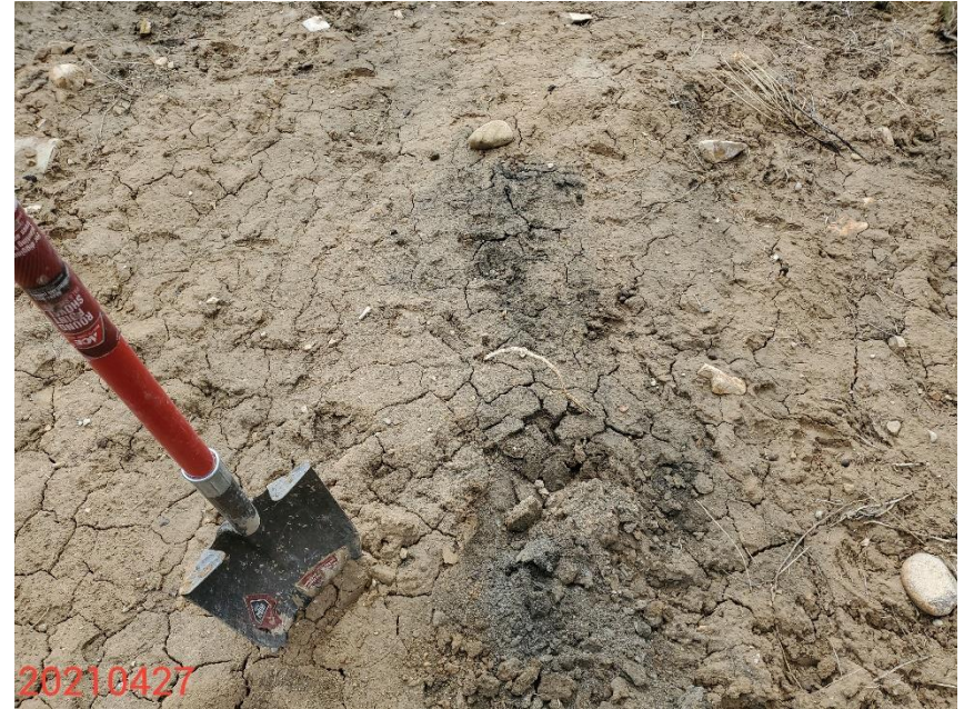
Photo 8: Photo shows areas where stained soils have not been removed.
