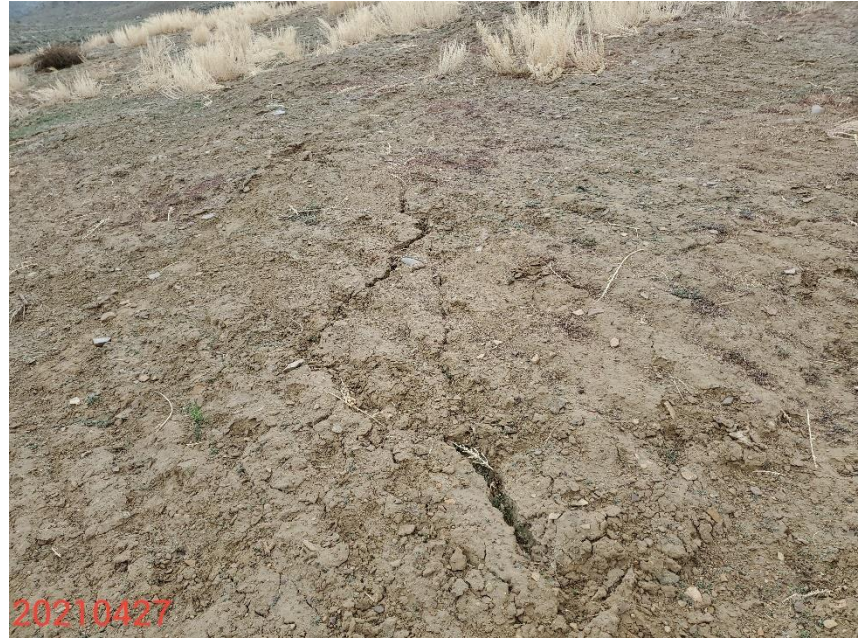
Photo 10: Previous inspections observed that stormwater erosion control BMPs were missing, or insufficient on the Location, and that cracking/rilling in soils were observed.
