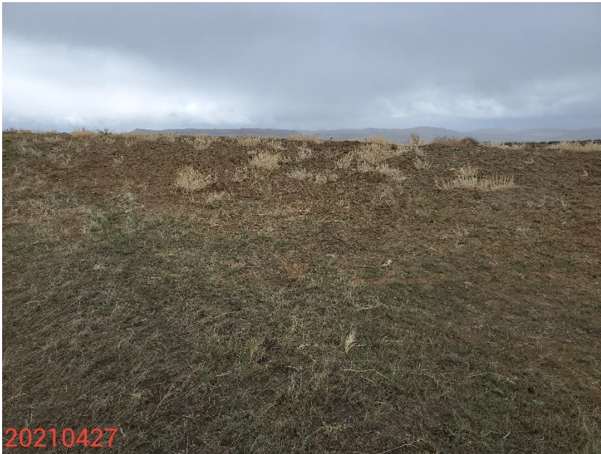
Photo 15: Photo taken from the southwest corner of the Location, facing north. Photo shows perimeter stormwater ditch. Ditch BMP has not been constructed in accordance with good engineering practices; BMP ends on the southwest end of the location and does not have a sufficient outlet to allow for sediment laden-free stormwater discharge.
