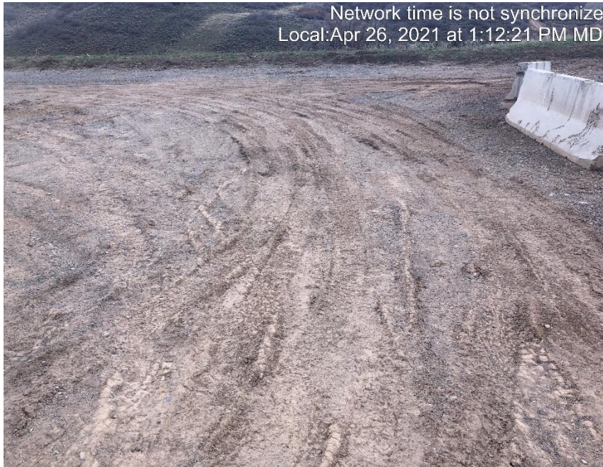
Photo #3622 Location lacks stabilization.
