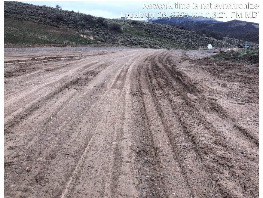
Photo #3623 no form of tracking BMP.
