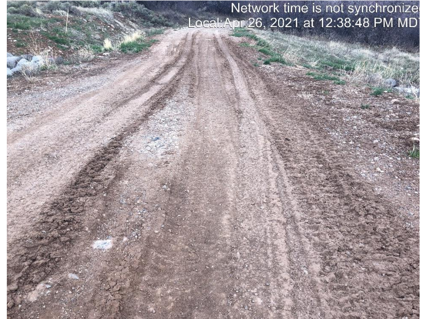
Photo #3619 No form of tracking BMP located at entrance to location.
