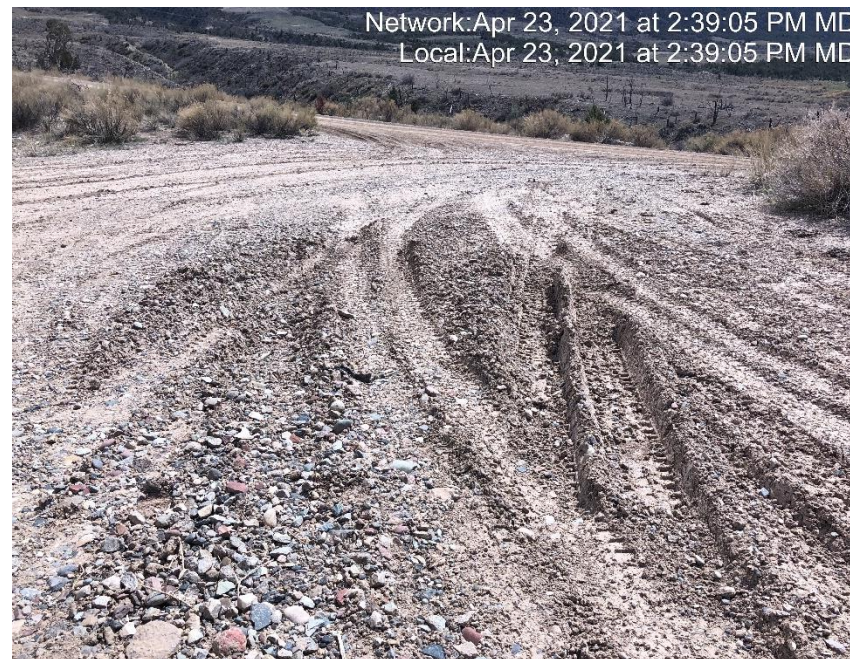
Photo #3614 No form of tracking BMP located at entrance to location.
