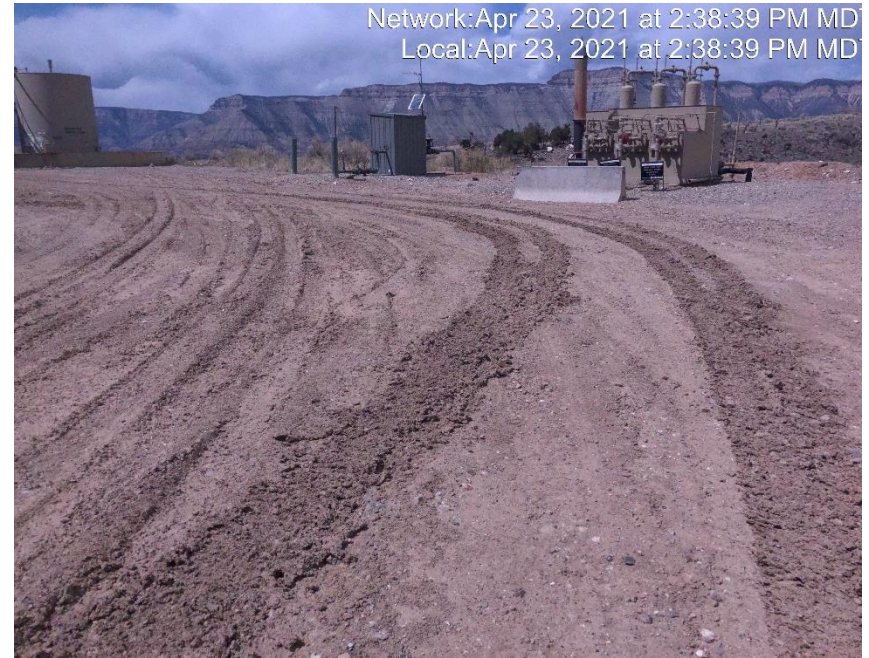
Photo #3616 location lacks stabilization.
