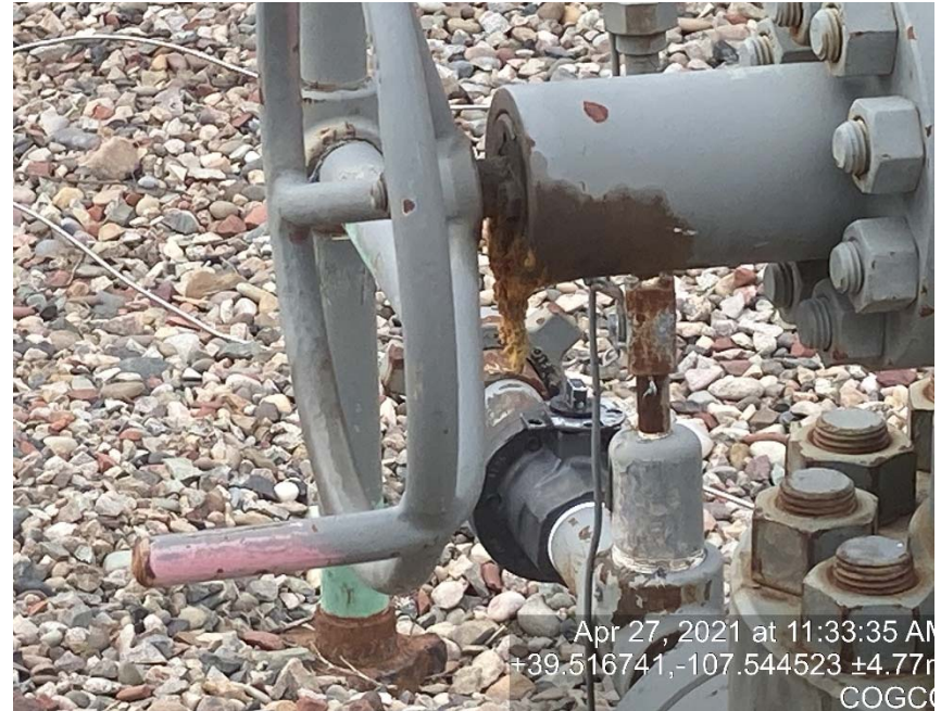
Master valve leaking
