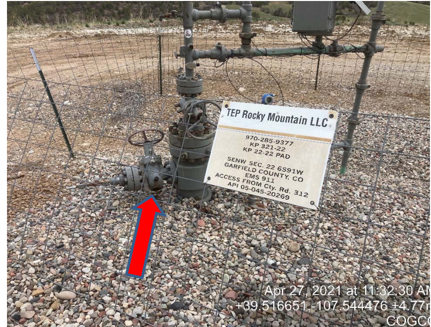
Grease Zurek leaking gas
