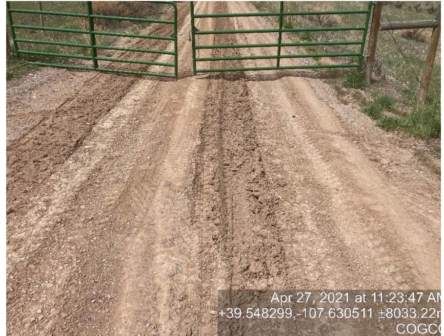
Lack of stabilization/compaction
