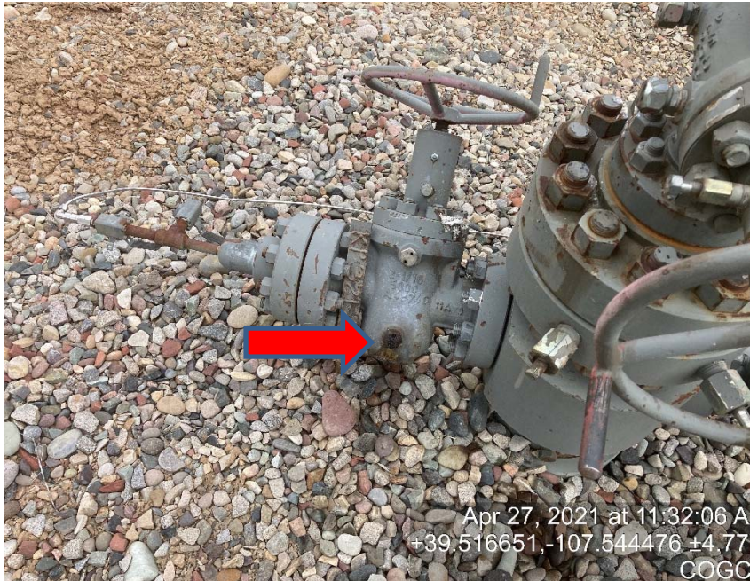
Grease Zurek leaking gas
