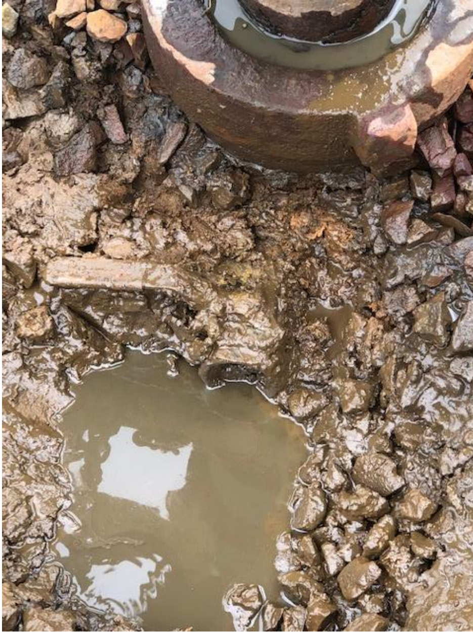
Plumbed Bradenhead to the surface to comply with Rule 341 and removed trash to comply with Rule 606.
