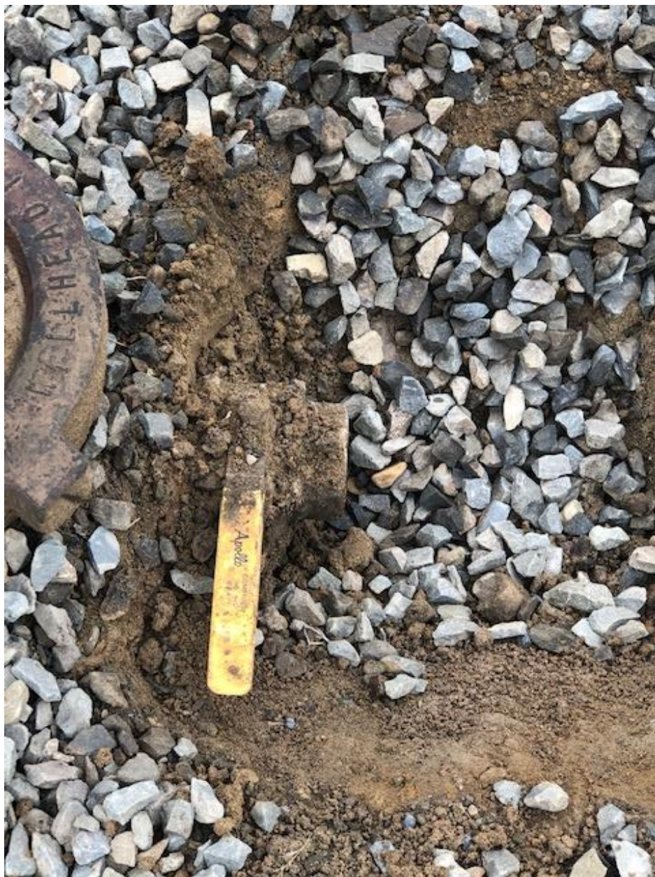
Plumbed Bradenhead to surface to comply with the new Rule 341.
