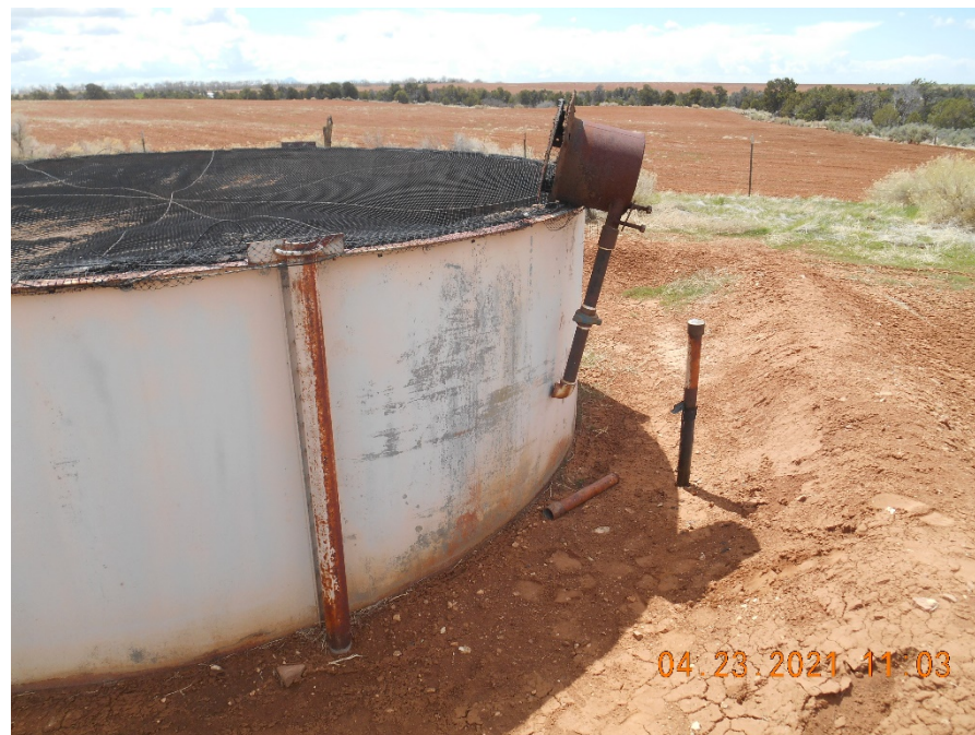
Broken elbow removed and flowline capped. CA completed.
