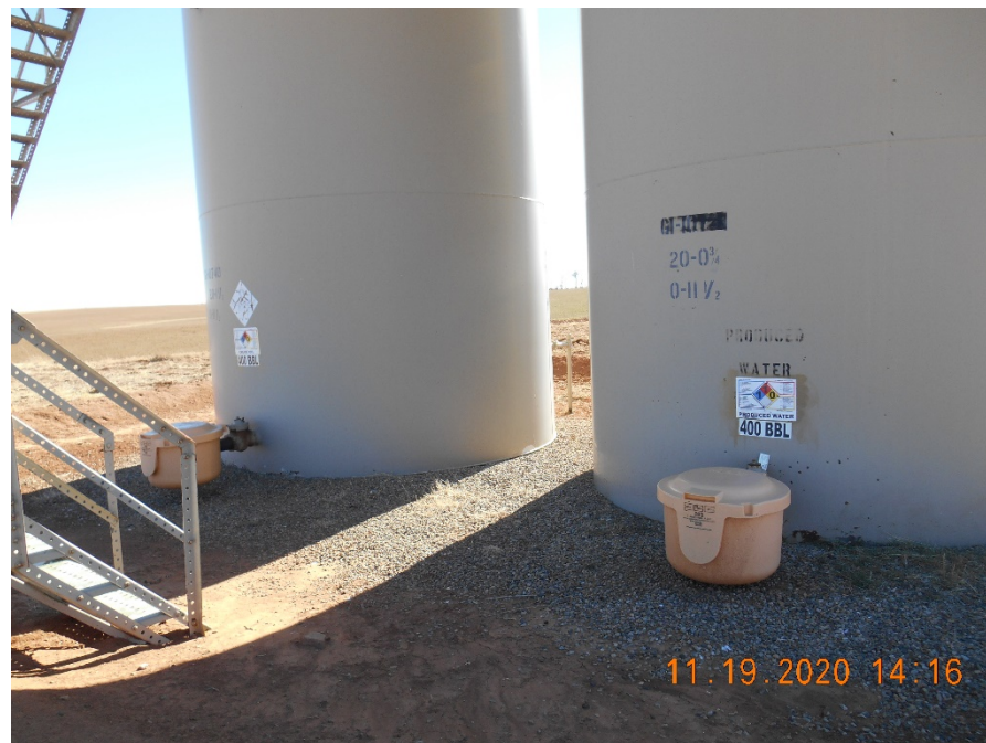
Improper tank labels.
