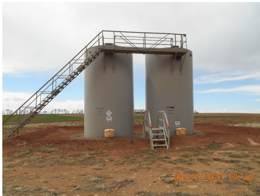
Tank battery with earth berms.
