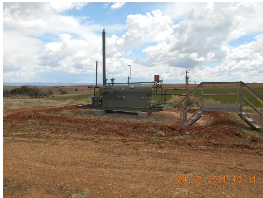
Separator with earth berms.
