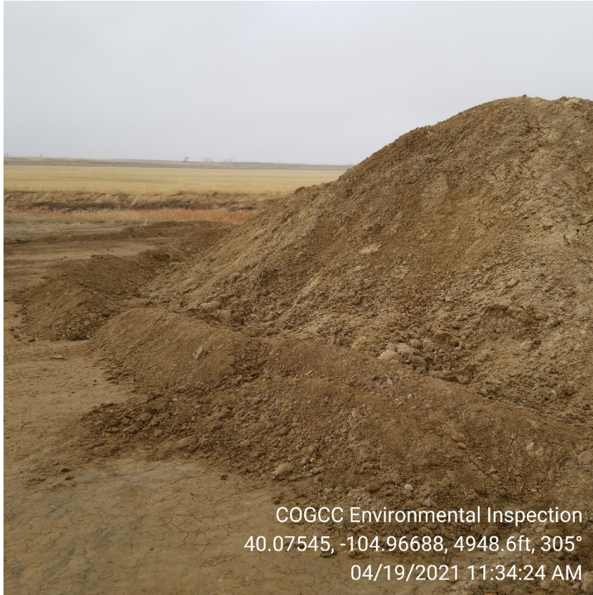
Photo 5 – Stockpiled soils with inadequate BMP's; wetland in background.
