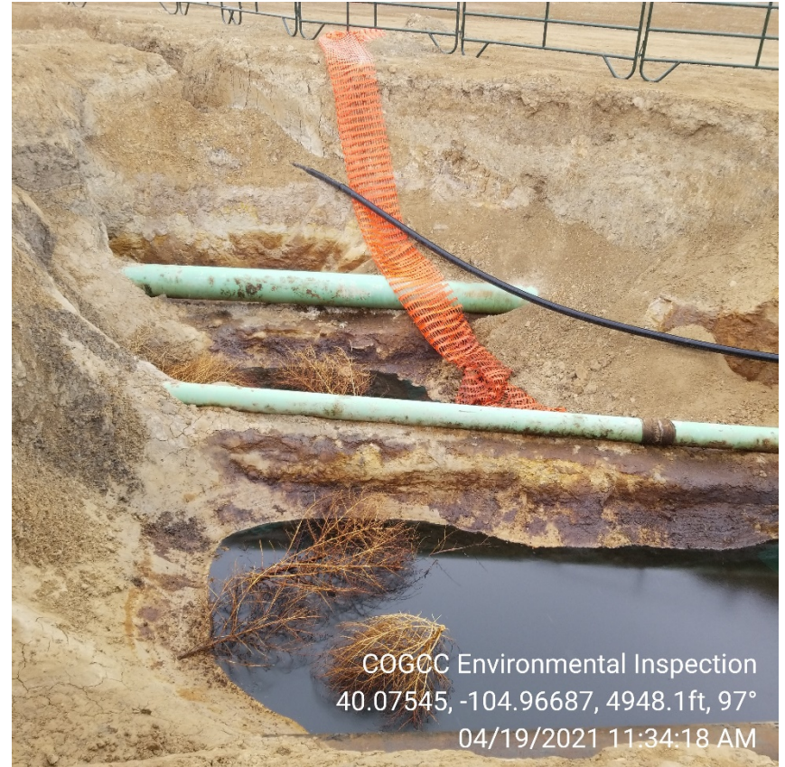
Photo 2 – Free product observed on groundwater. Flowlines exposed and trash in excavation.
