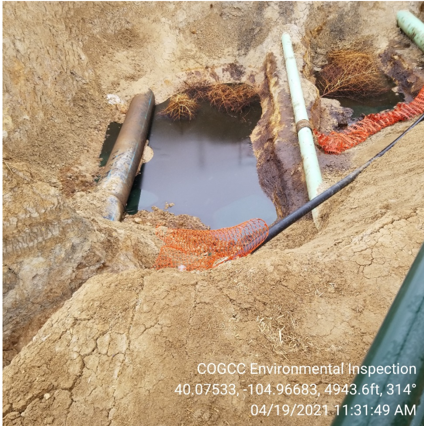
Photo 1 – Free product observed on groundwater. Flowlines exposed and trash in excavation.
