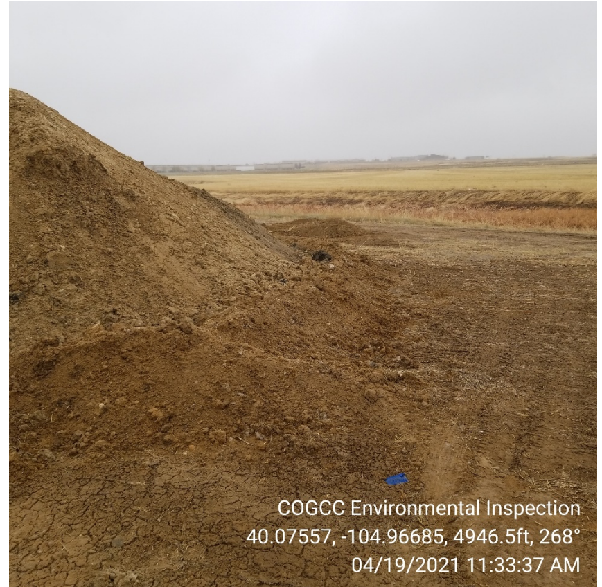
Photo 6 – Stockpiled soils with inadequate BMP's; wetland in background.
