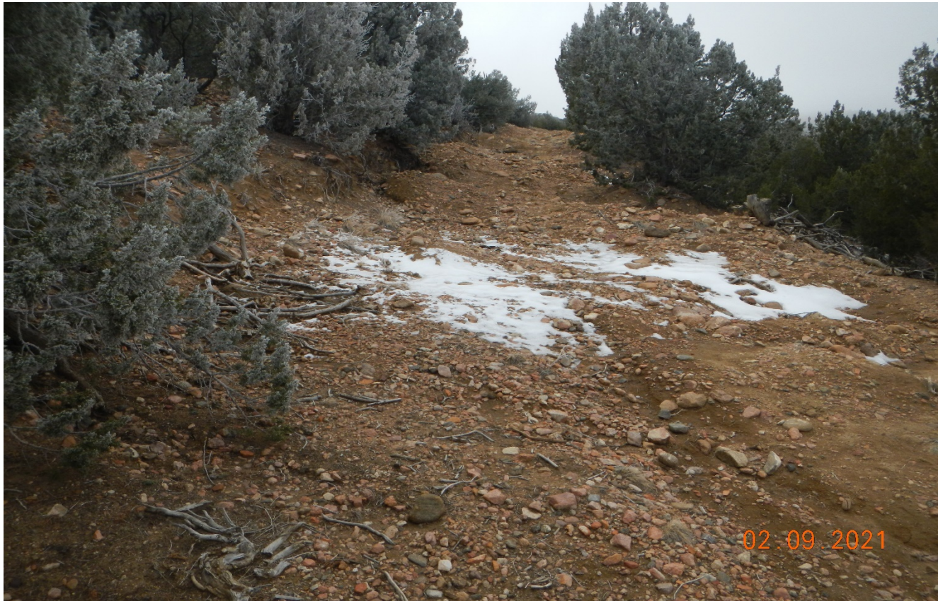
Photo 4. Facing southwest along the access road between the Hassler 24 and Drapper4 well site. This area has not been recontoured and reclaimed and is susceptible to further erosion.
