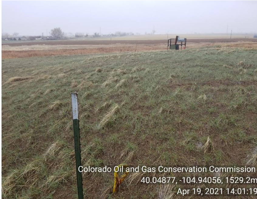
Photo 3 Guy line anchors not properly marked.
