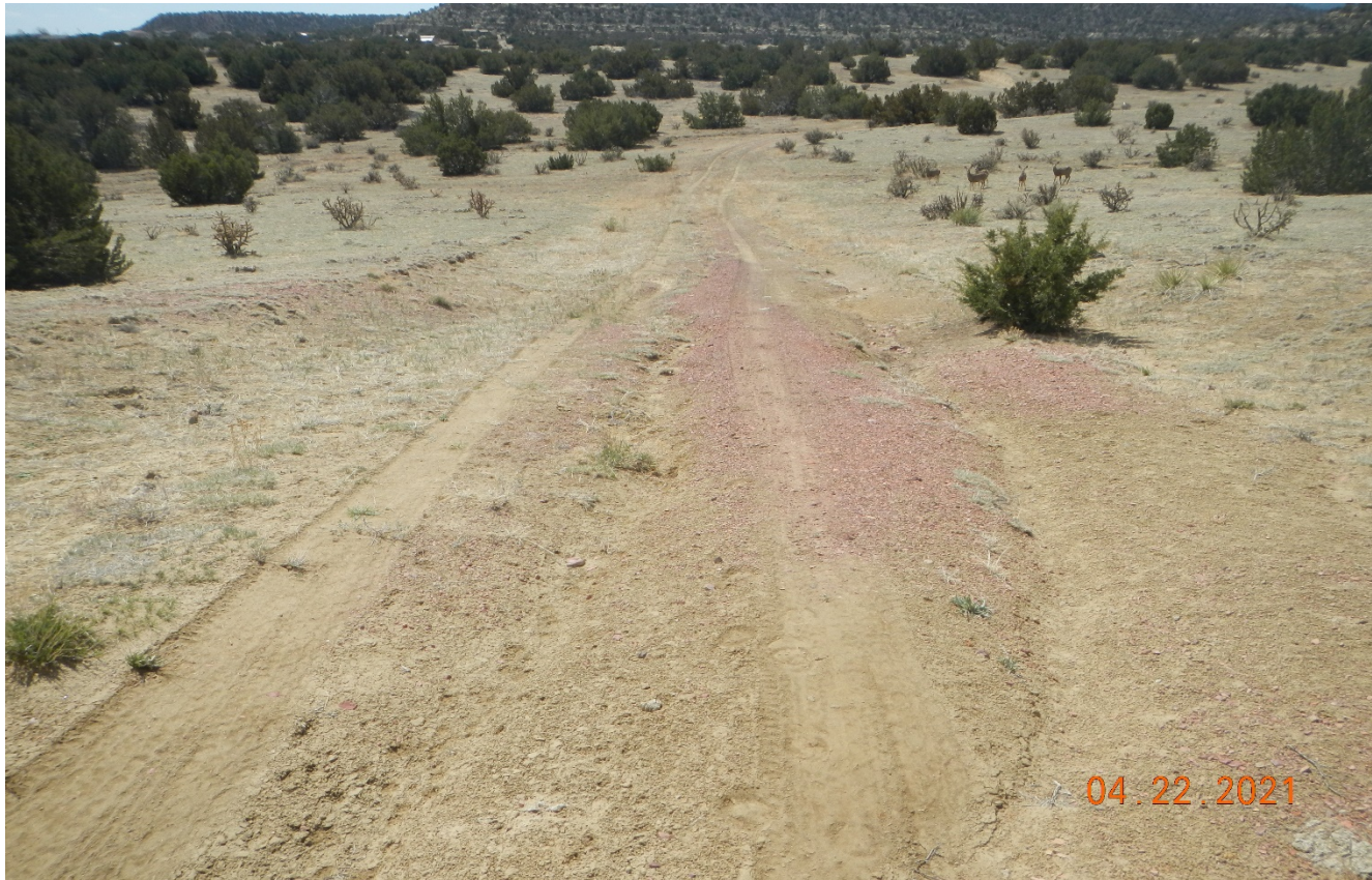
Photo 1. Facing south along the main access road. There is erosion along this area of the road which needs to be repaired and stabilized.
