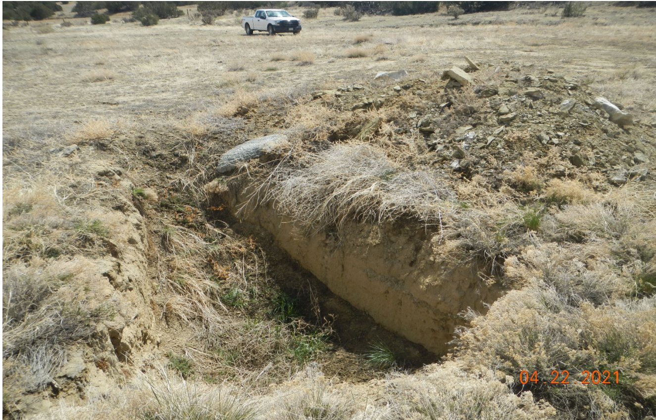
Photo 5. There is an open hole which is about 4.5 ft. deep. There is cement debris next to the hole which appears to be from plugging of the well.
