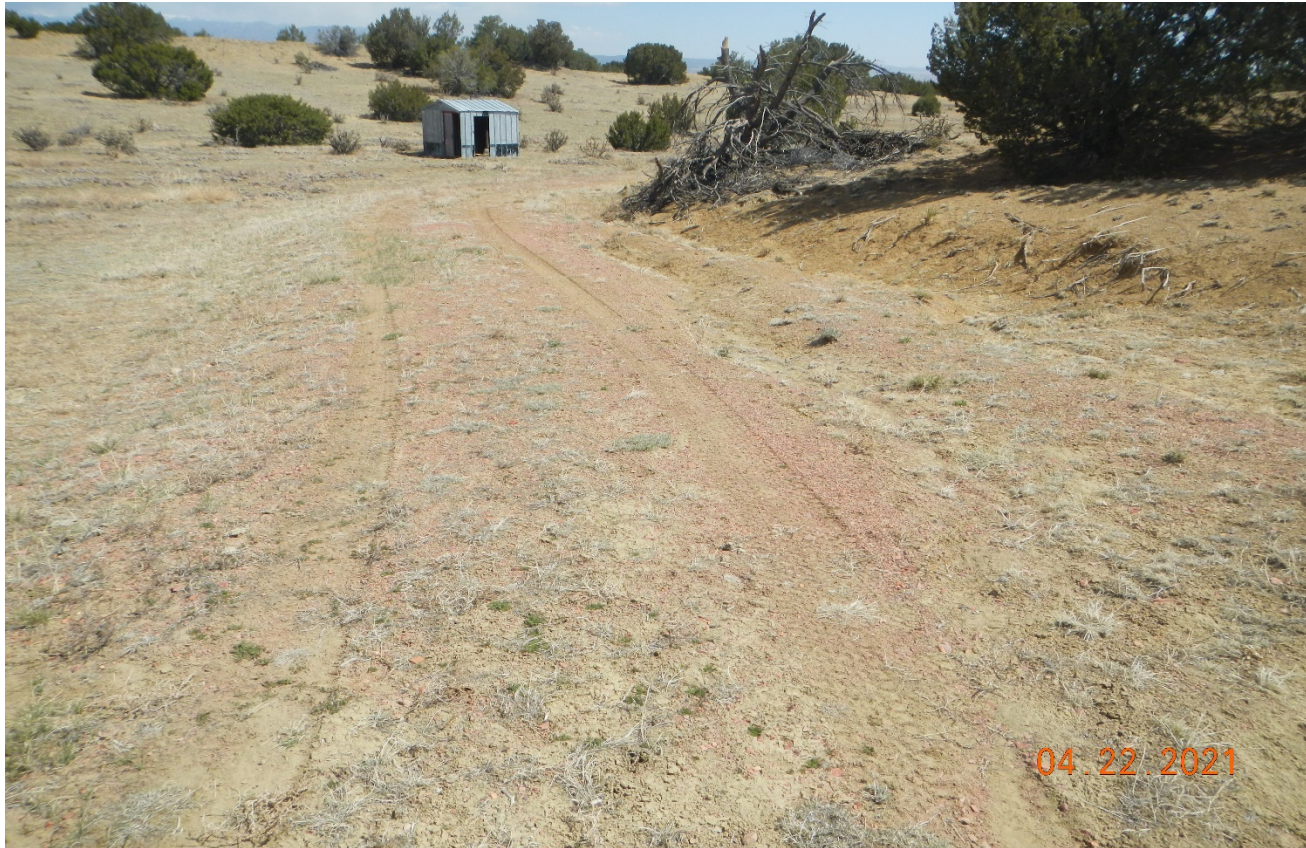
Photo 2. Facing northeast along the access road. The access road has not been recontoured and reclaimed.
