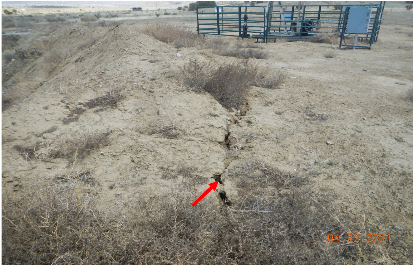
Photo 7. This crack in the soil surface near the well is an indication of potential soil sloughing. This area needs to be stabilized.
