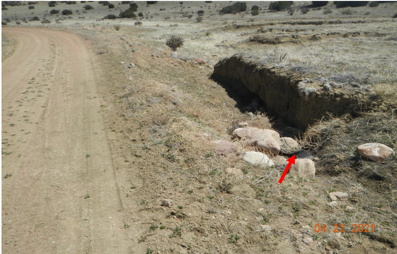
Photo 1. Facing east along the access road. The gully erosion along the road has not been repaired and stabilized. There is a tire placed in gully shown at red arrow which needs to be removed. A few rocks scattered in the gully is insufficient stabilization.
