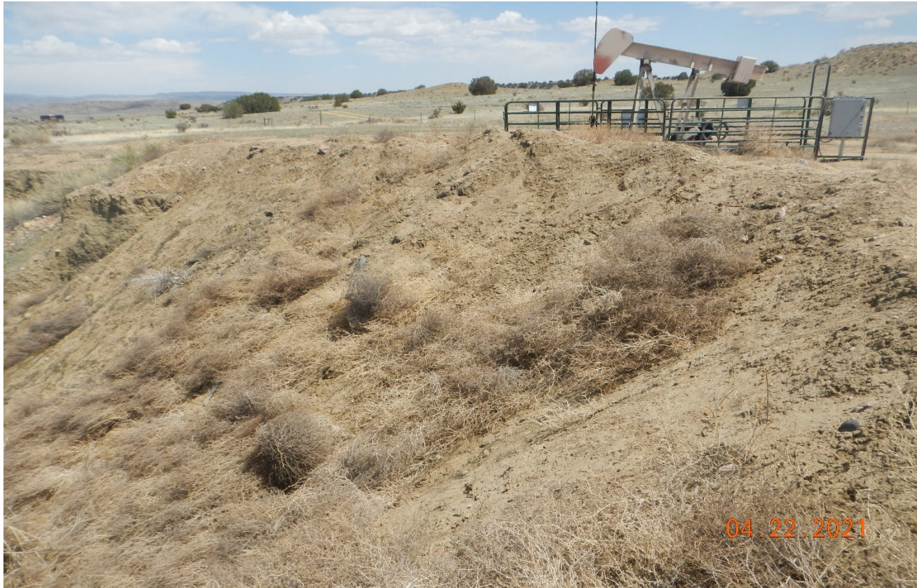
Photo 6. Facing northwest toward the embankment near the well. This area has not been stabilized.
