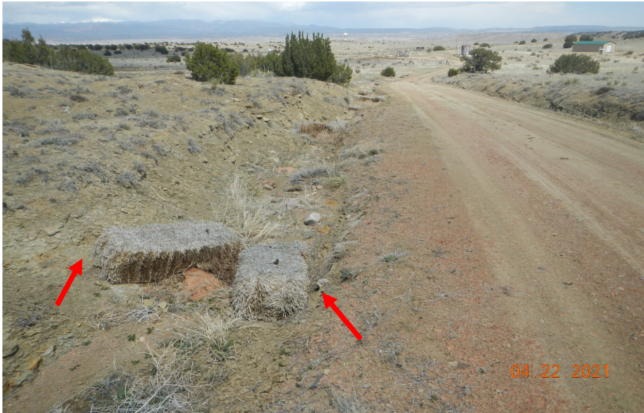
Photo 2. Facing northeast along the access road where erosion is occurring along the road. There are straw bales that are placed along the side of the road which are insufficient. Stormwater can flow around the bales show at red arrows.
