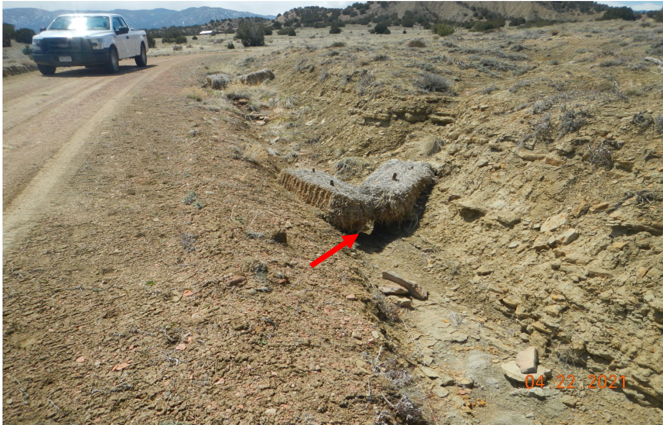
Photo 3. The bales are not installed correctly and stormwater is causing erosion underneath the bales which essentially is not working.
