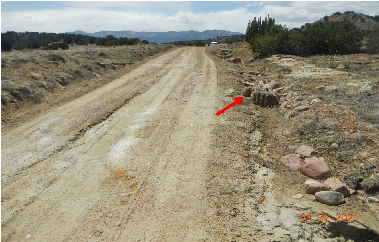
Photo 4. Facing southwest along the road. This straw bales is displaced. Stormwater erosion is not controlled along the roadside.
