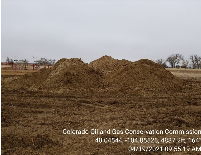
Photo 5 – Soil stored on location with inadequate BMPs.
