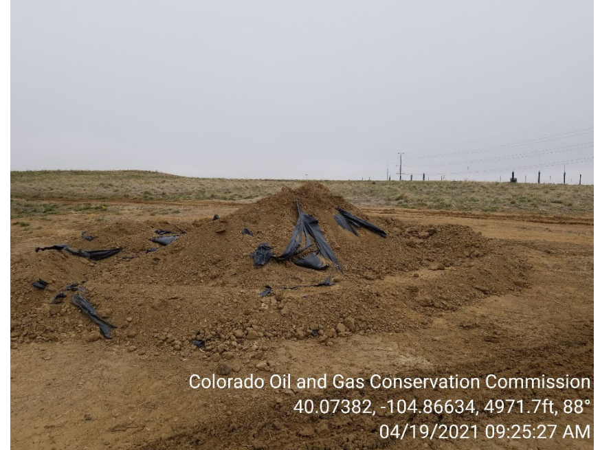
Photo 8 – Oily soils stockpiled on location. Lining not present under the entirety of soils pile.
