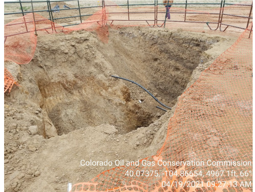
Photo 4 – Open excavation. Impacts remain in situ. Trash observed in excavation.
