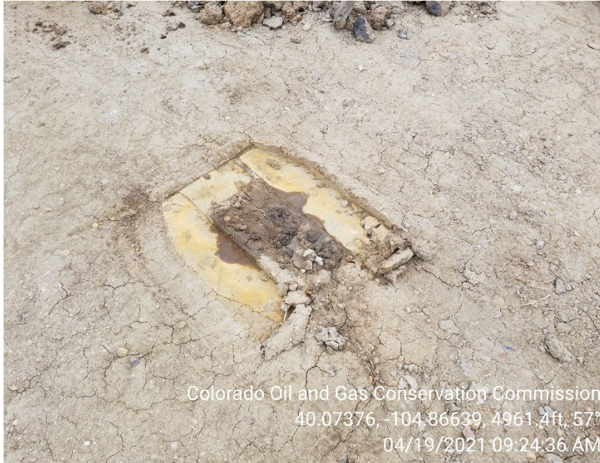
Photo 9 – Stained soil observed around open excavation.
