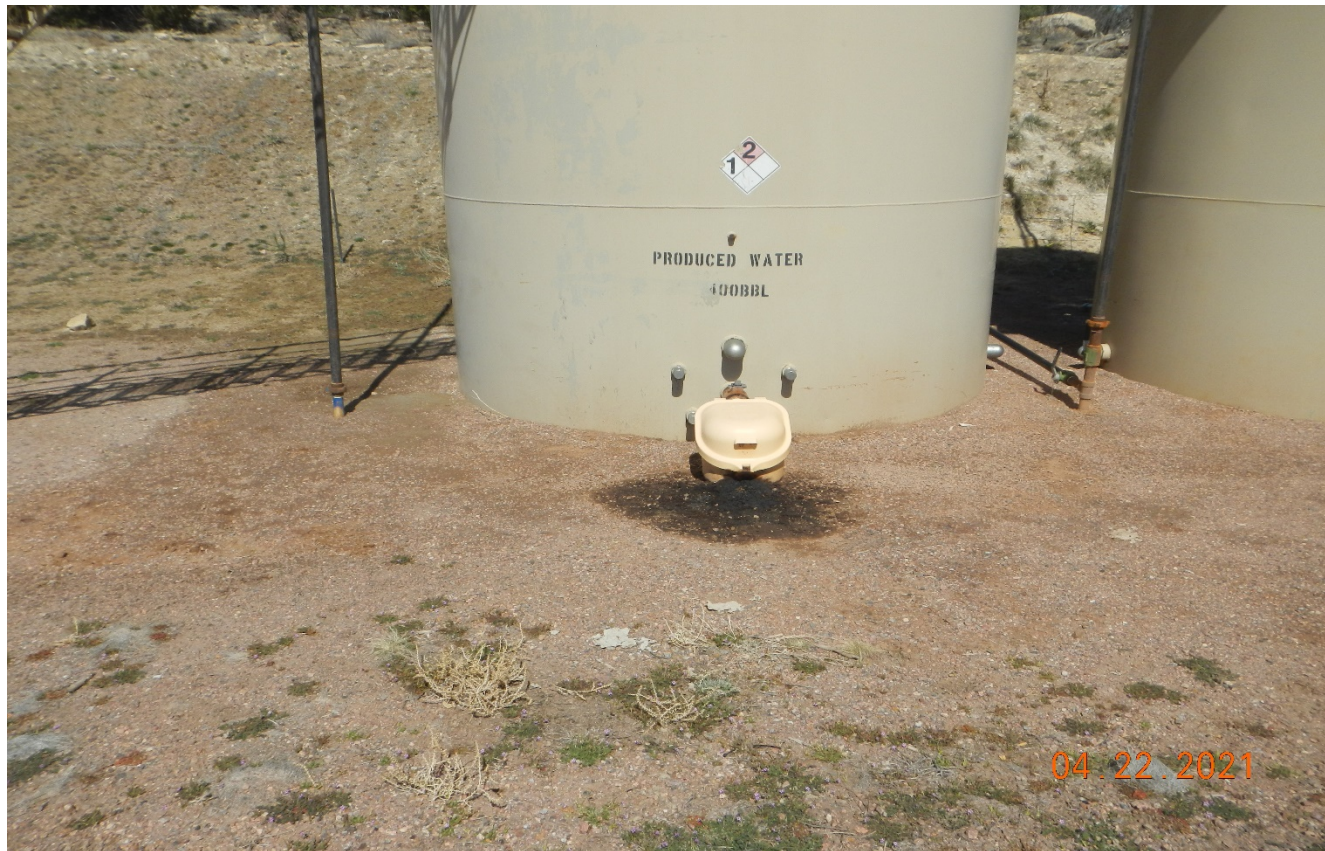
Photo 9. There is stained soil at the outlet of the PW tank.
