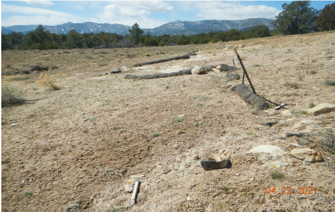
Photo 5. There are wattles displaced at the southwest side of the location. Wattles need to be repaired and maintained. Previous corrective action has not been performed.
