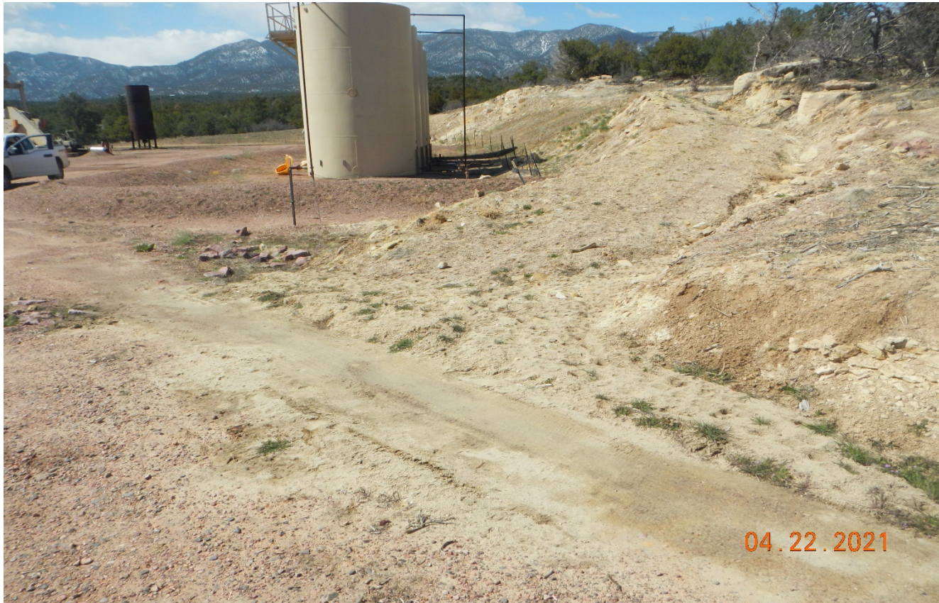
Photo 10. The top perimeter ditch is directing stormwater toward the road which has deposited sediment onto the road. BMP's are needed in this area. Previous corrective action has not been performed.
