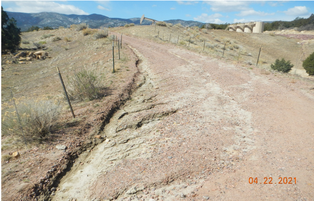
Photo 2. There is erosion along the access road. Stormwater is diverted down the road and into drainage area shown in previous photo. The erosion needs to be repaired and stormwater needs to be properly diverted. Previous corrective action has not been performed.
