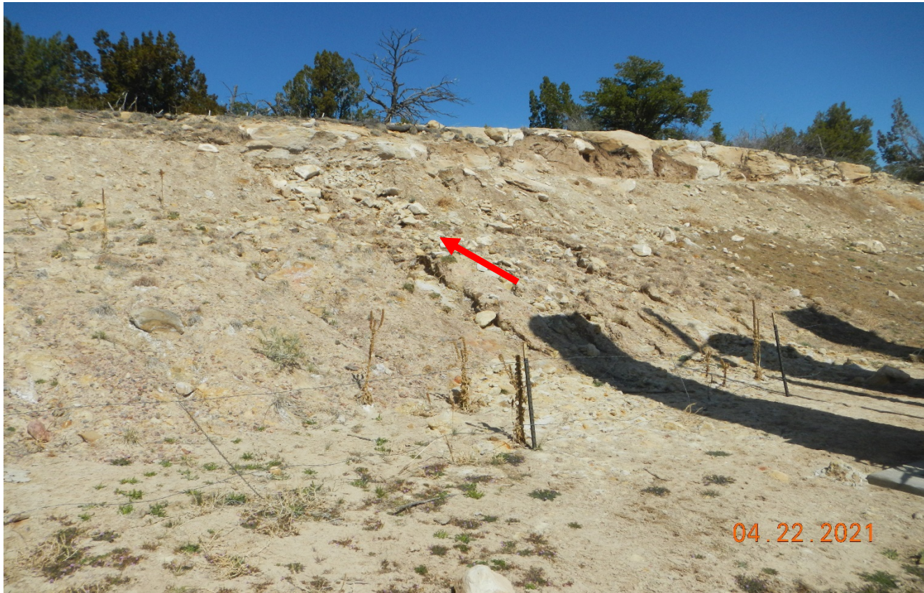
Photo 7. There is an erosion occurring off the cut slope.
