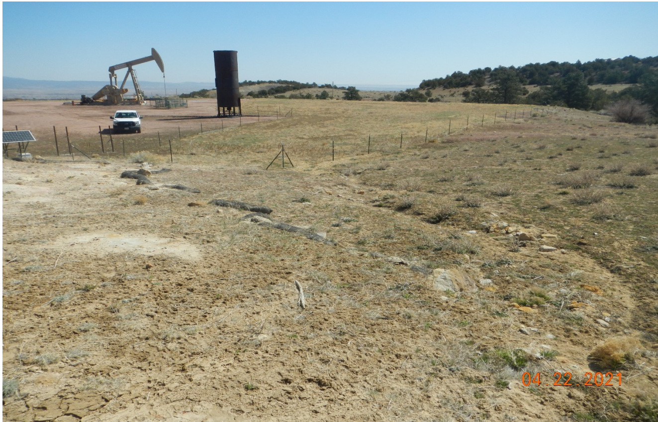
Photo 6. There is an erosion channel at the southwest side of the location. Stormwater is directed to this area from the top perimeter ditch. BMP's are needed in this area to prevent erosion.
