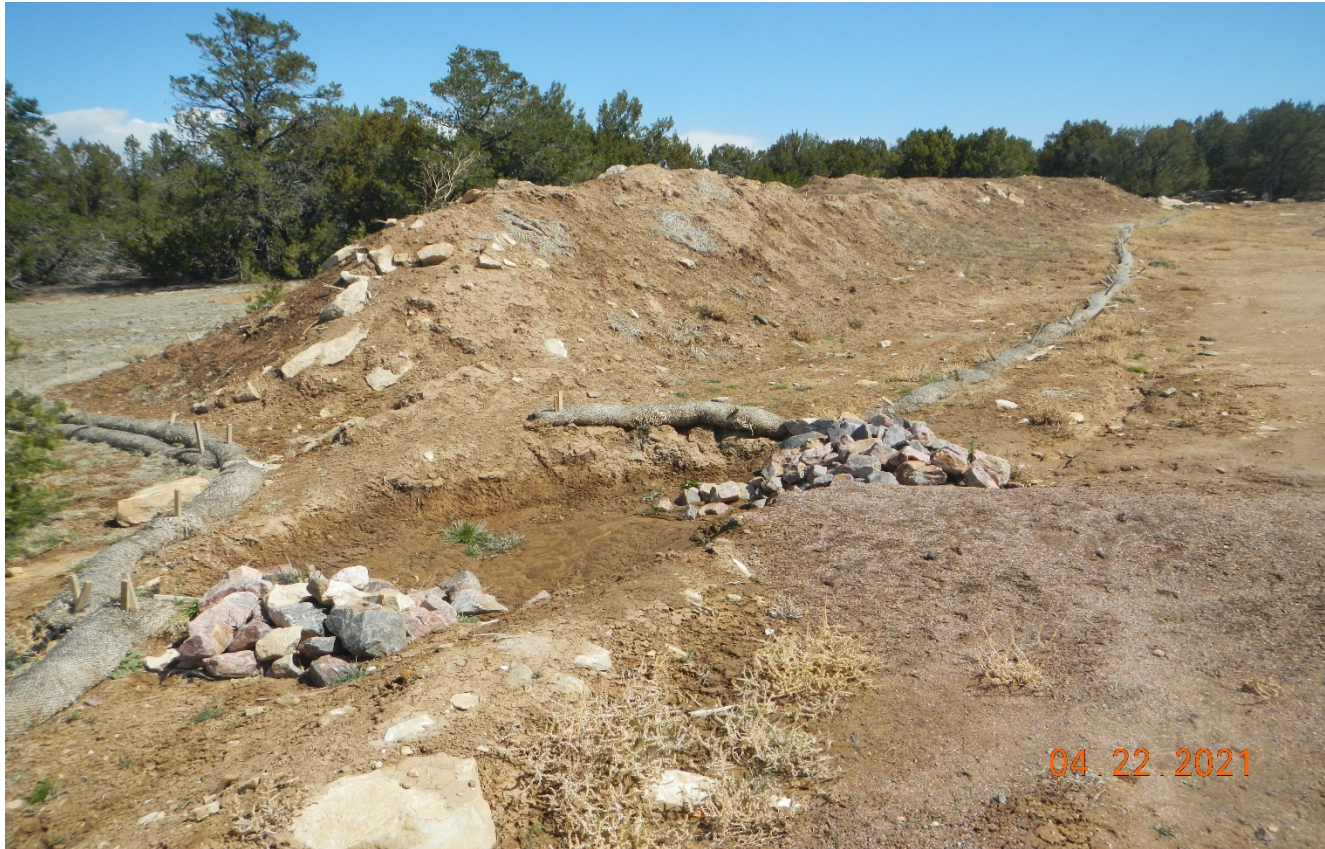
Photo 11. Facing northwest toward the topsoil pile which are not maintained and protected from degradation and weed infestation. Previous corrective action has not been performed. The BMP's around the stockpile are not maintained.
