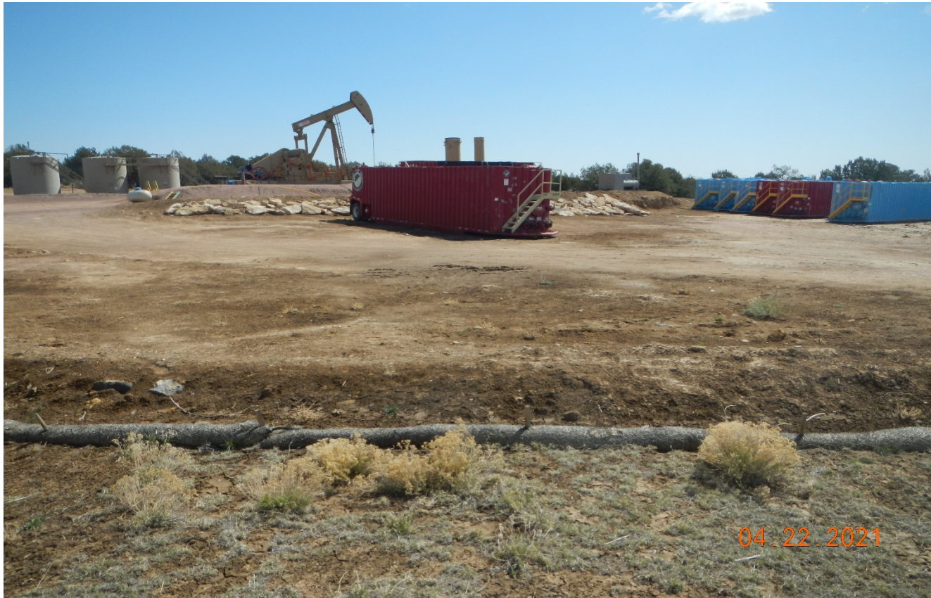
Photo 12. Facing northeast toward the location. The unused tanks need to be removed. Unused areas of the location need to be recontoured and reclaimed. Previous corrective actions have not been performed.
