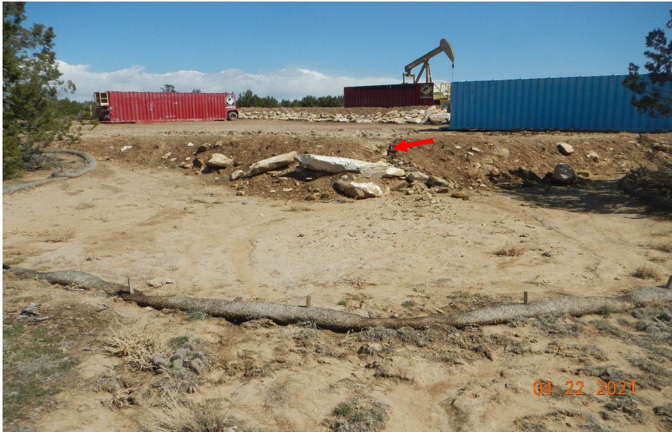
Photo 3. Facing north at the south corner of the location. There is erosion occurring from the disturbed pad site which is filling in the perimeter wattles. Previous corrective action has not been performed.
