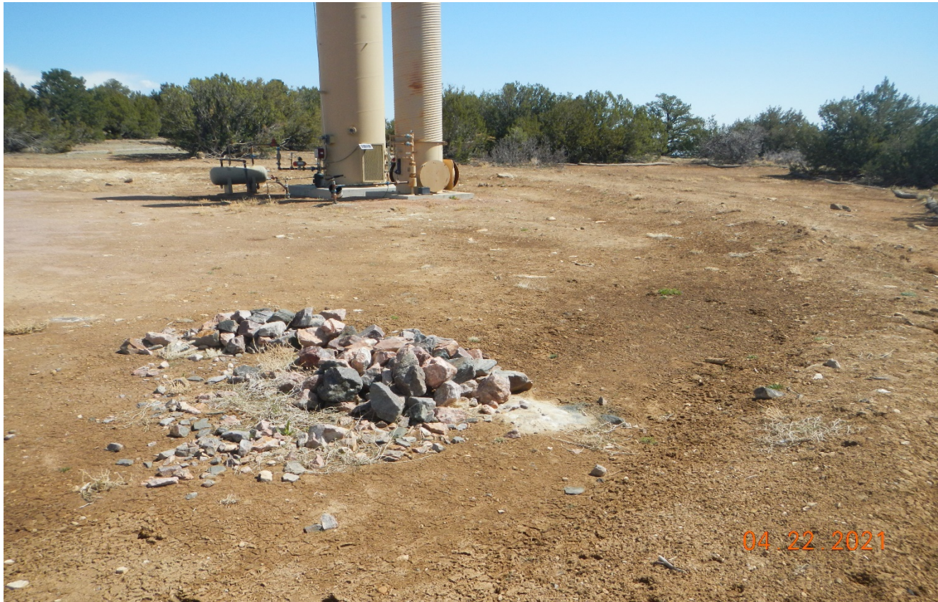
Photo 5. Facing north at the location. Disturbed areas around the location have not been reclaimed and stabilized. A pile of rock debris remains in this area.
