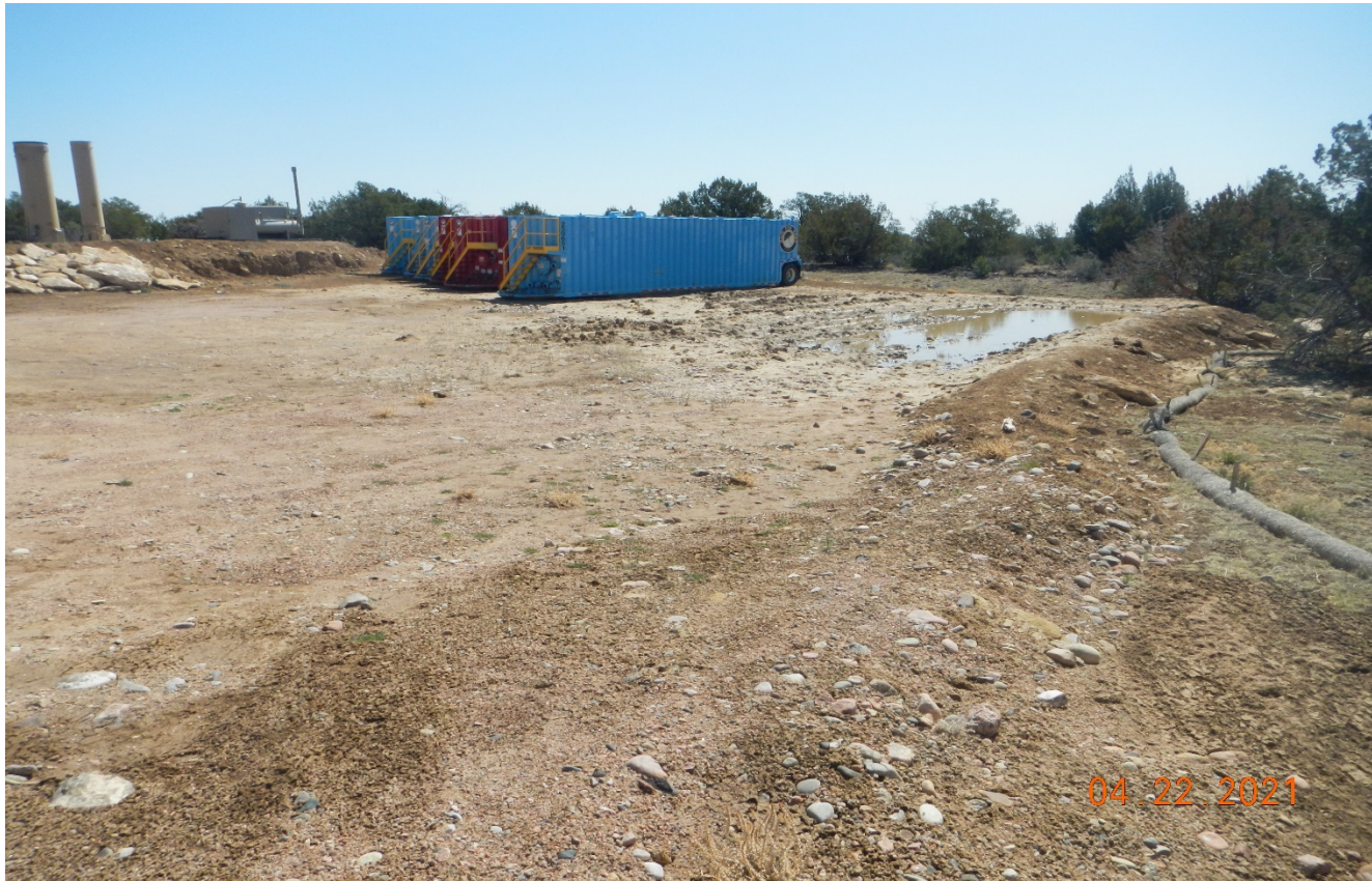
Photo 2. Facing east at the location. There is 5 frac tanks staged that remain at east side of the location. The tanks have not been removed since previous inspection. Previous corrective actions have not been performed.
