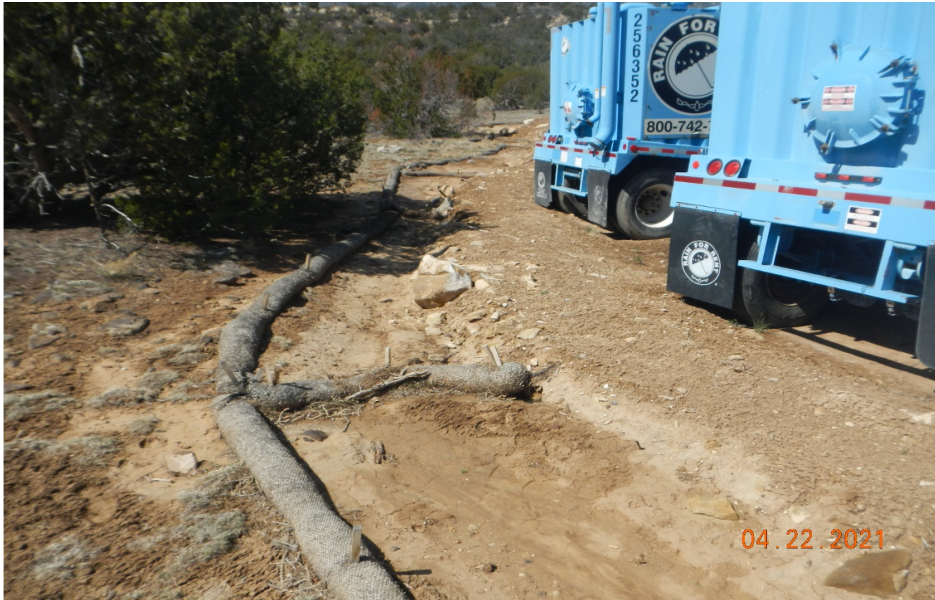
Photo 4. Facing southwest behind the frac tanks. The wattles have filled in with sediment. Previous corrective action has not been performed.
