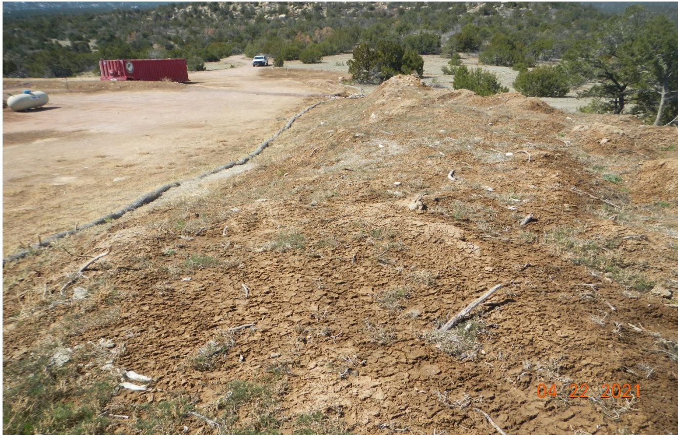
Photo 10. Facing toward the topsoil pile. The topsoil piles are not stabilized and protected. Topsoil piles have not been replaced for interim reclamation. There are undesirable weeds germinating on the stockpiles.
