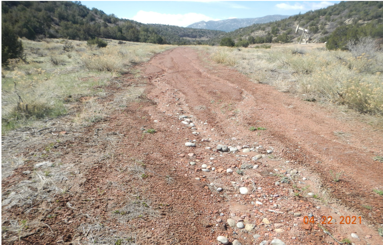
Photo 1. Facing south along the access road. There is erosion occurring down the road which needs to be repaired and stormwater needs to be diverted off the road. Previous corrective action has not been performed.
