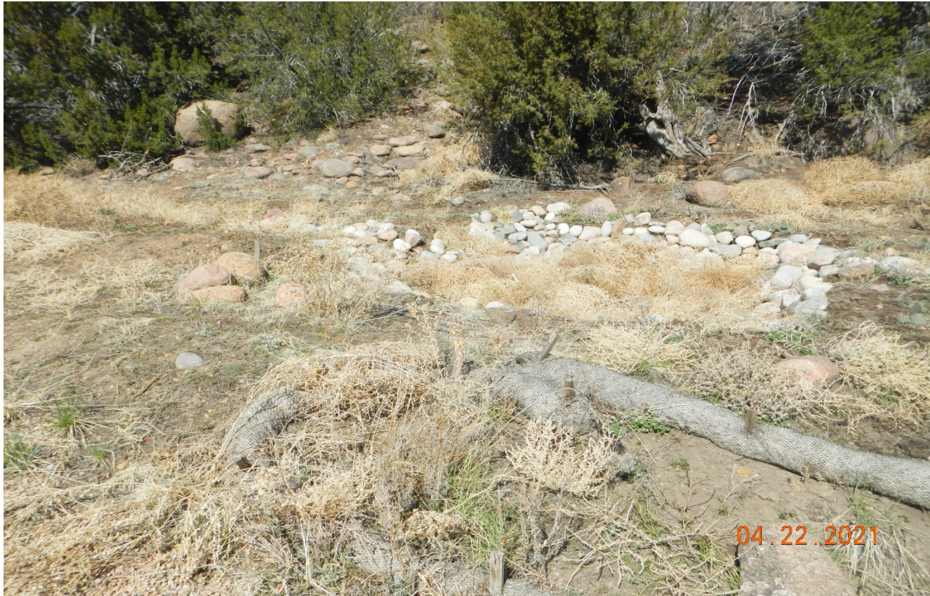
Photo 9. Facing toward the sediment trap. Undesirable weed debris needs to be removed out of sediment trap.
