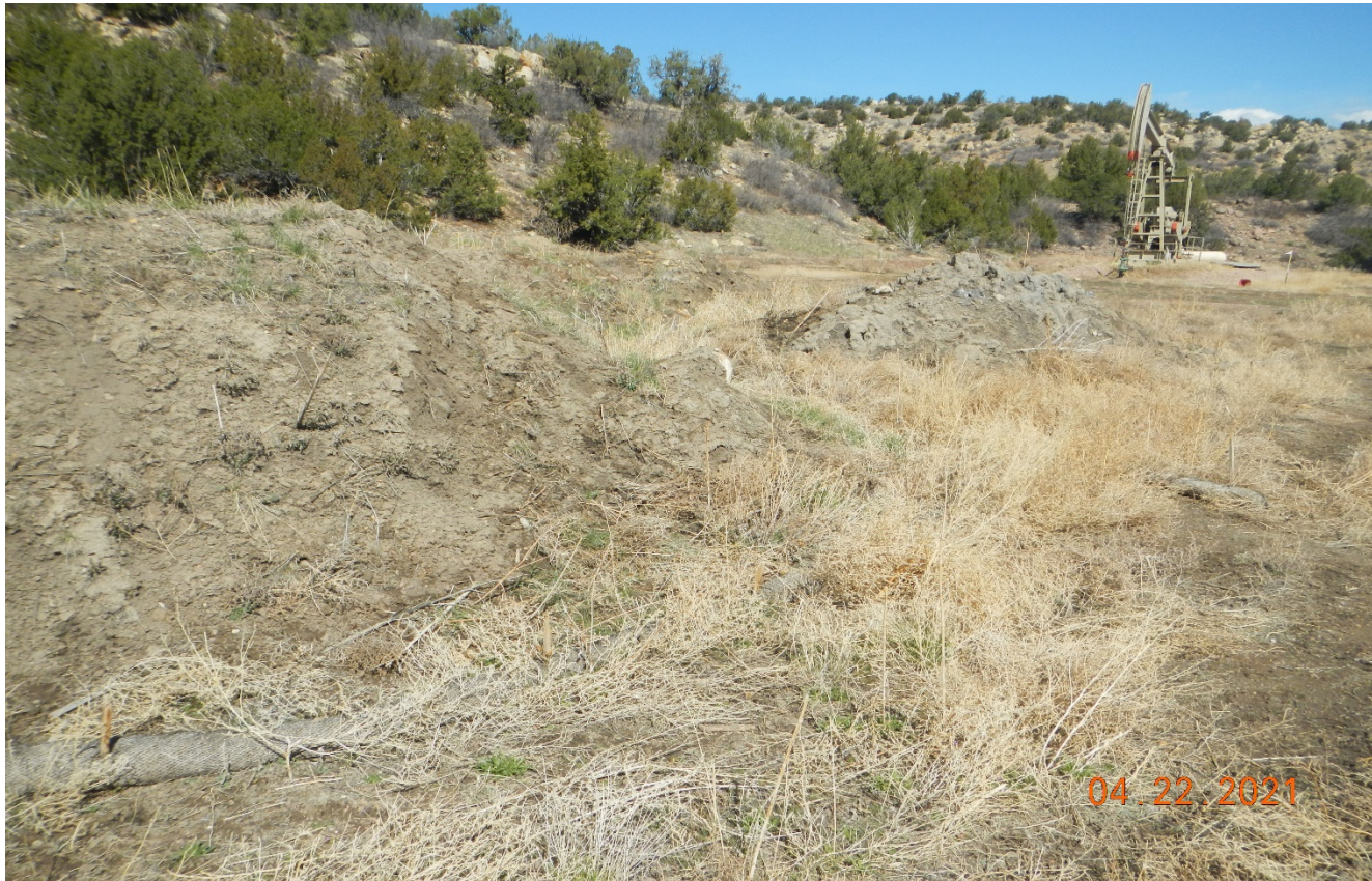
Photo 5. The soil piles are not maintained and have undesirable weeds. The soil piles need to be replaced for interim reclamation. Previous corrective action has not been performed.
