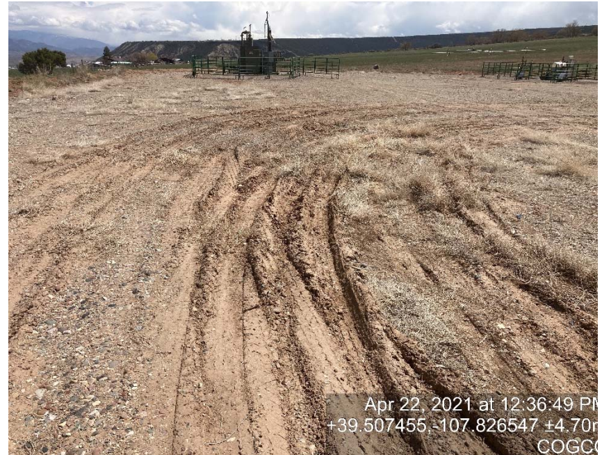
Lack of stabilization/compaction
