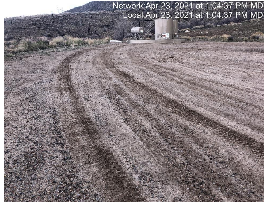
Photo #3601 Location lacks stabilization
