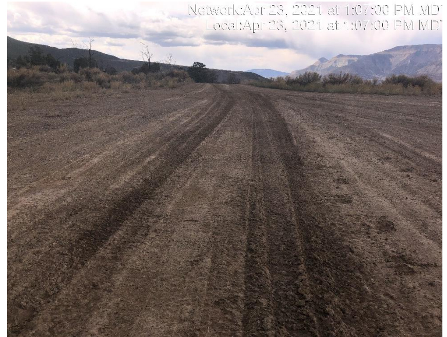
Photo #3604 No form of tracking BMP at entrance to location.
