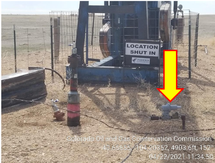
Photo 3 – Wellhead – Unmarked Riser, Weeds
