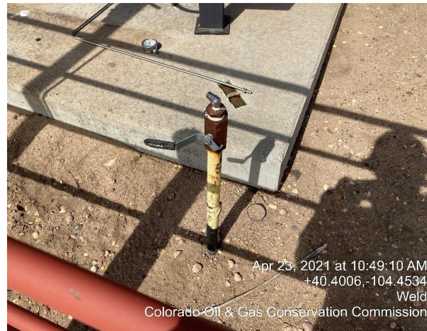
Photo #4 Riser not marked or locked out
