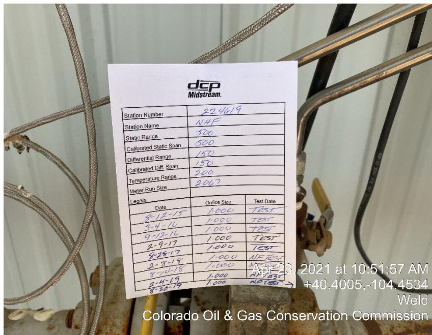
Photo #5 Not updated calibrated gas meter
