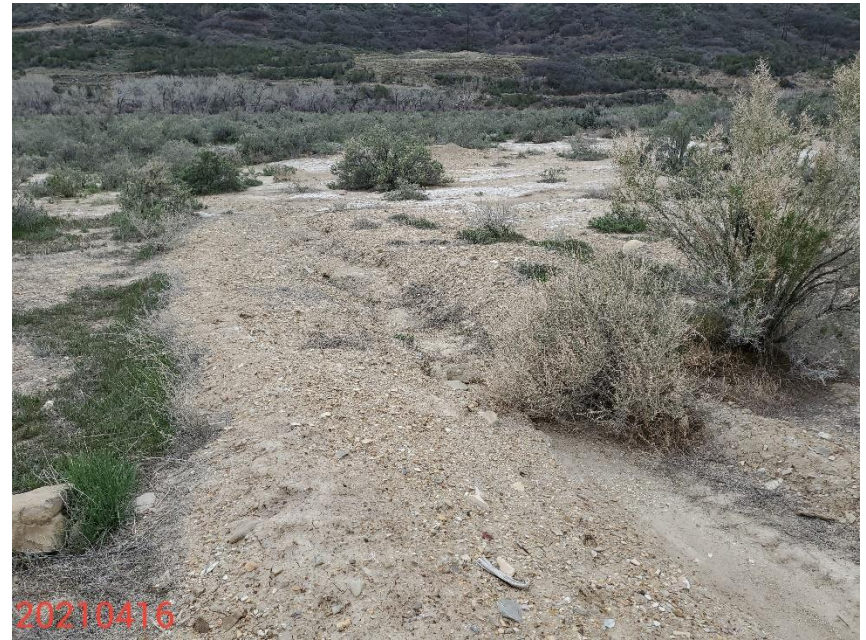
Photo 4: Photo taken from the south end of the Location, facing south. Photo shows erosion degradation on interim areas due to stormwater runoff from the Location and access road; stormwater and erosion control measures on the Location missing or insufficient.
