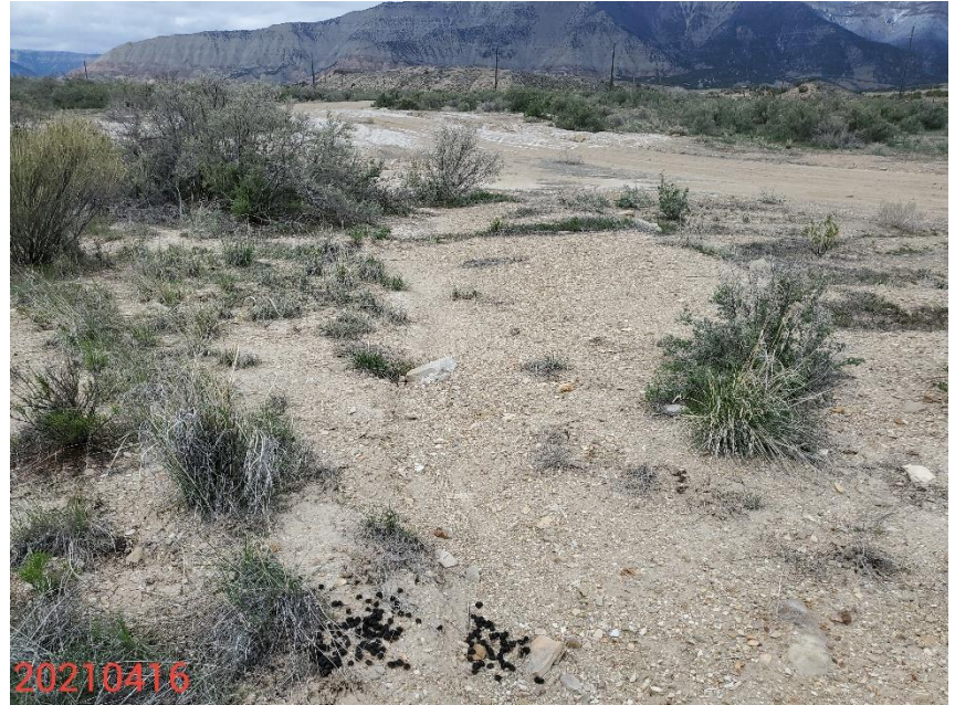
Photo 10: Photo taken from the interim areas on the southwest end of the Location, facing northwest. Photo shows erosion degradation and sediment deposition from stormwater runoff. Additional reclamation required.
