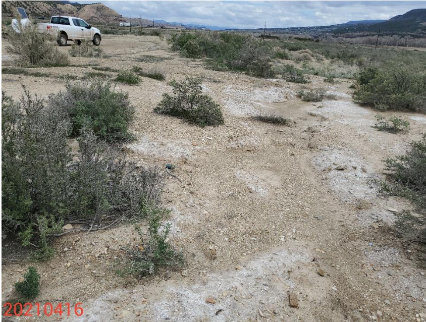
Photo 9: Photo taken from the interim areas on the southwest end of the Location, facing east. Photo shows erosion degradation and sediment deposition from stormwater runoff. Additional reclamation required.
