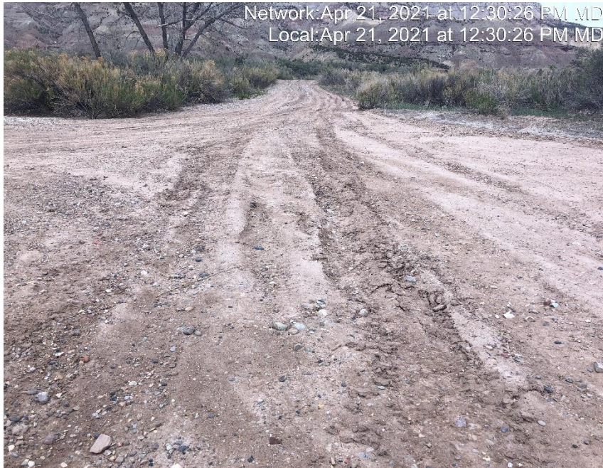
Photo #3576 No form of tracking BMP located at entrance to location.
