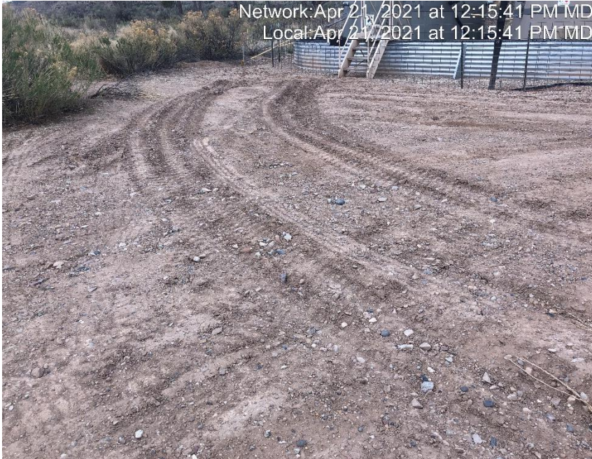
Photo #3574 Location lacks stabilization.
