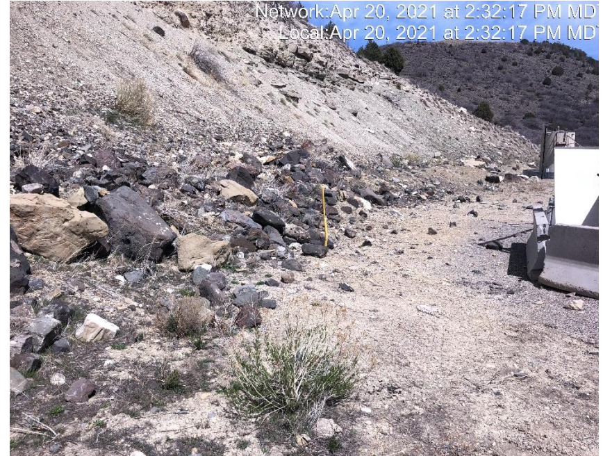
Photo #3568 Cut slope lacks stabilization
