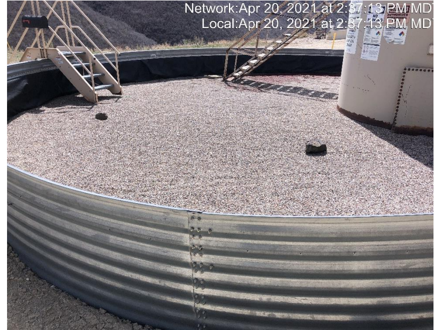
Photo #3570 Rocks and debris are encroaching on production equipment.
