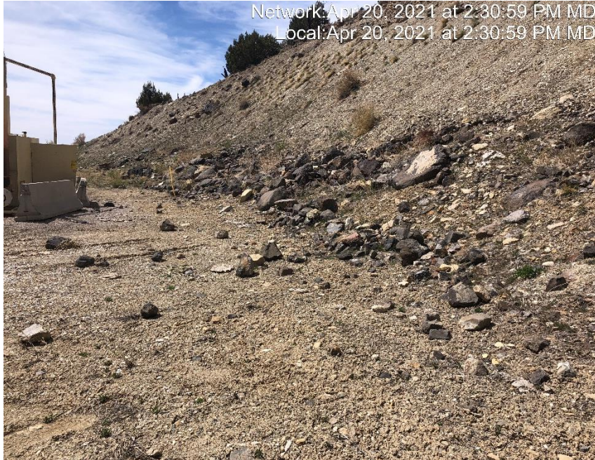
Photo #3567 Cut slope lacks stabilization
